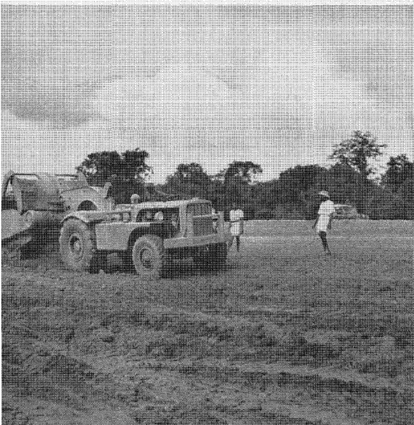
This Caterpillar tractor is hauling fill dirt for airport construction on the Gal Oya project. The Ceylonese were trained as drivers.
