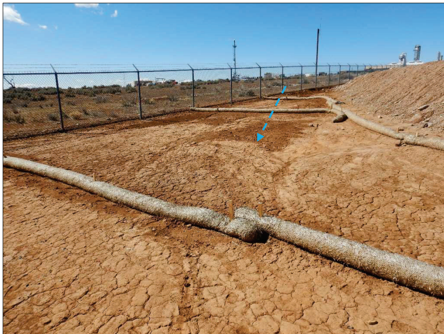
Photograph 106. Additional view, facing Southwest, of straw wattles along fence line in Drainage Area 15, near the Soil Drying Containment Area, downgradient from the area shown in Photograph 105. Note sediment accumulation against the wattles.
