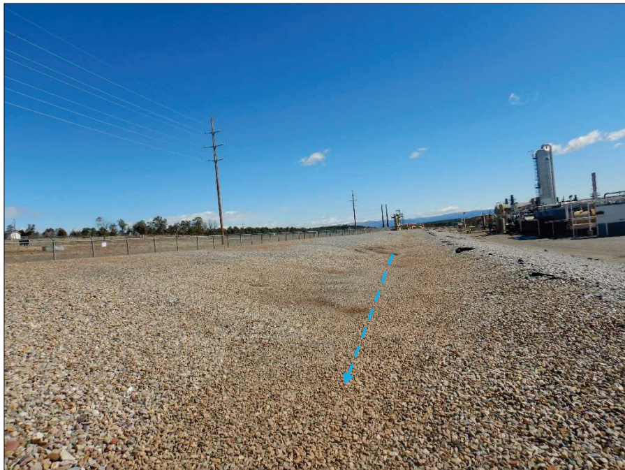
Photograph 70. View, facing East, of ditch along northern fence line of Facility that drains to Outfall IGP-001.
