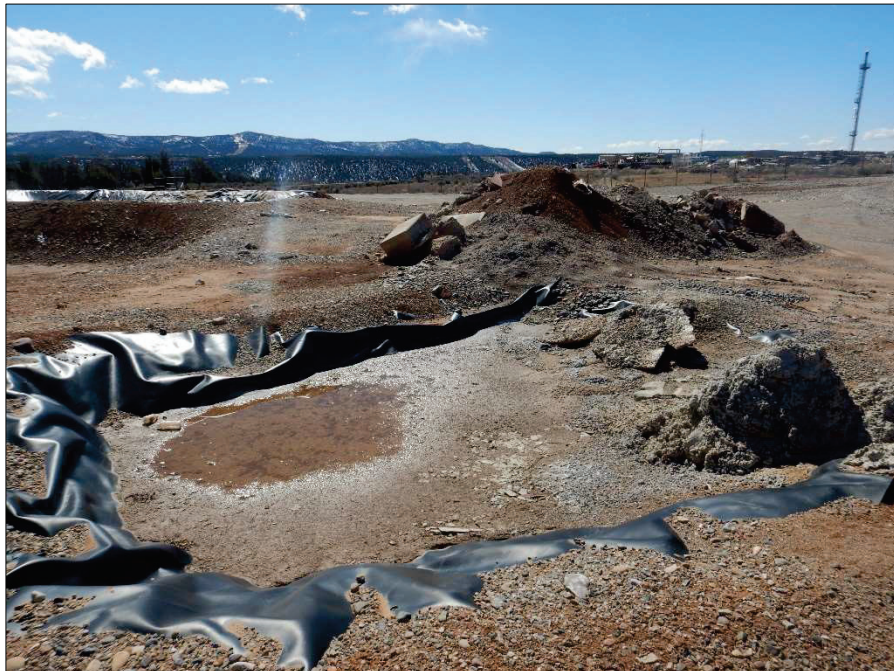
Photograph 112. View, facing Southwest, of a concrete washout area located in Drainage Area 15. The concrete wash out area was more than half full at the time of the inspection.
