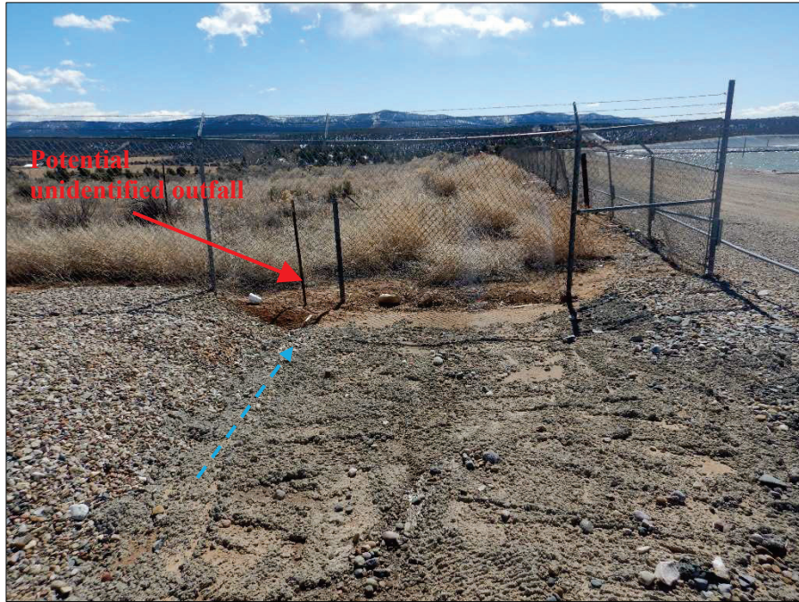
Photograph 21. View, facing South, of a potential unidentified outfall in Drainage Area 14.
