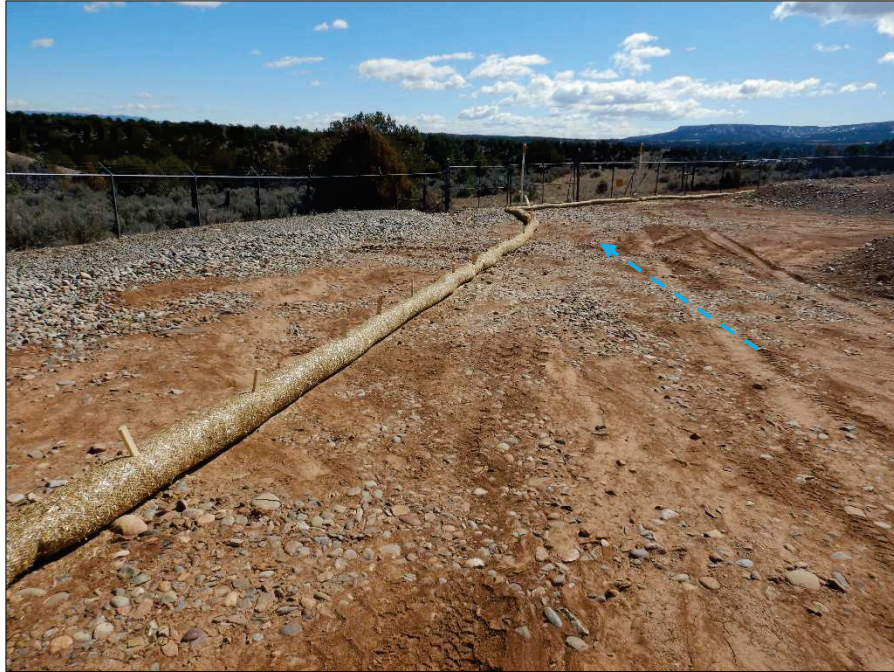
Photograph 107. View, facing Southeast, of new straw wattles near Outfall IGP-004.
