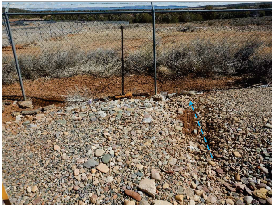
Photograph 16. Additional view, facing East, of the stormwater drainage pathway leading from the Facility's boneyard toward the potential unidentified outfall shown in Photograph 25, as referenced in Photograph 15.
