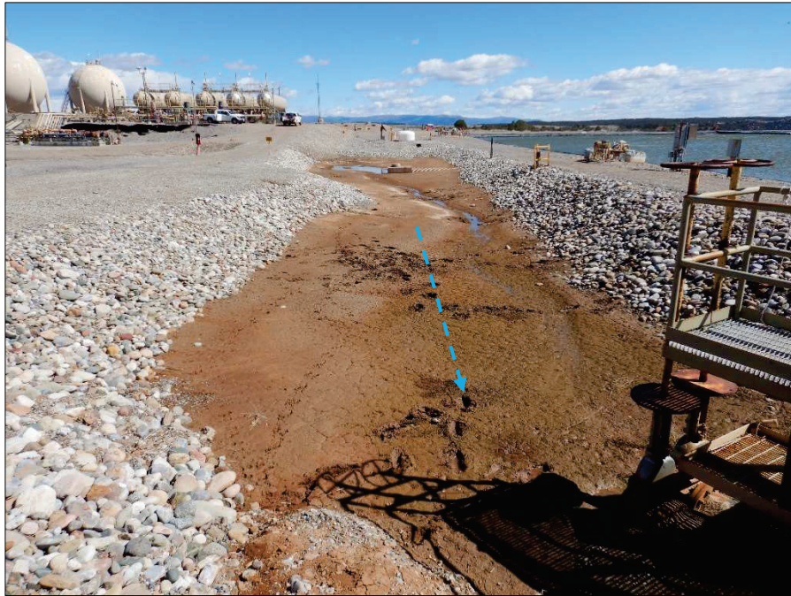
Photograph 53. View, facing East, of North Evaporation Stormwater Holding Pond. Note sediment accumulation in the pond.
