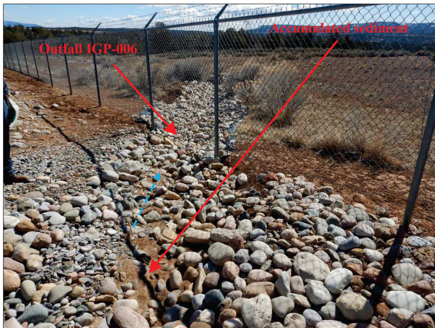
Photograph 94. View, facing Southeast, of Outfall IGP-006. Note accumulated sediment upgradient from the outfall.
