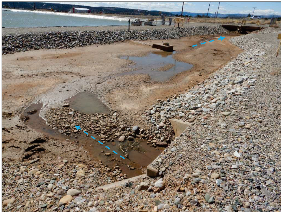
Photograph 56. Additional view, facing Southwest, of North Evaporation Stormwater Holding Pond, as referenced in Photographs 53 through 55. Note sediment accumulation in the pond.
