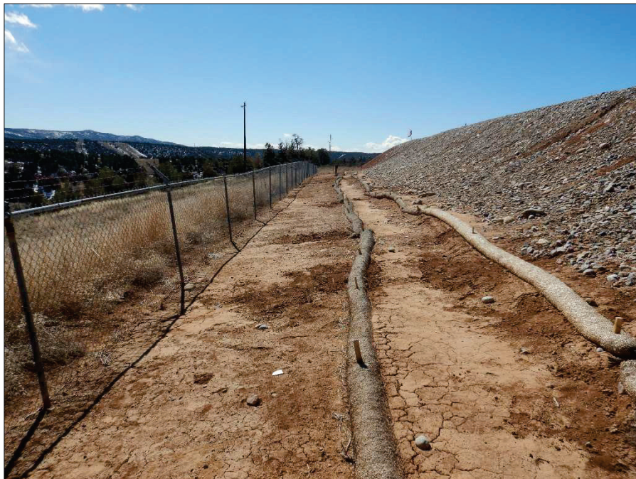
Photograph 110. View, facing Southwest, of straw wattles along the southeastern side of South Evaporation Pond. Note sediment accumulation against the wattles.
