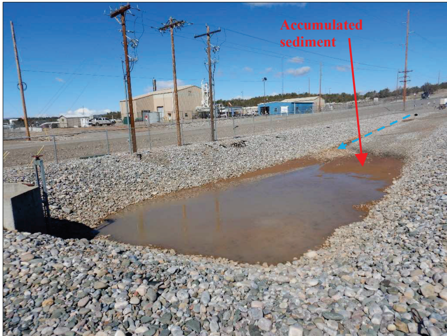
Photograph 64. View, facing Northwest, of Gosney Pond. Note accumulated sediment in the pond.
