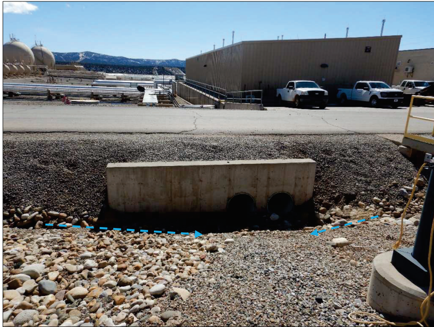
Photograph 51. Additional view, facing South, inlet of culvert and ditch near parking lot connecting to the ditch leading to North Evaporation Stormwater Holding Pond, as referenced in Photograph 50.
