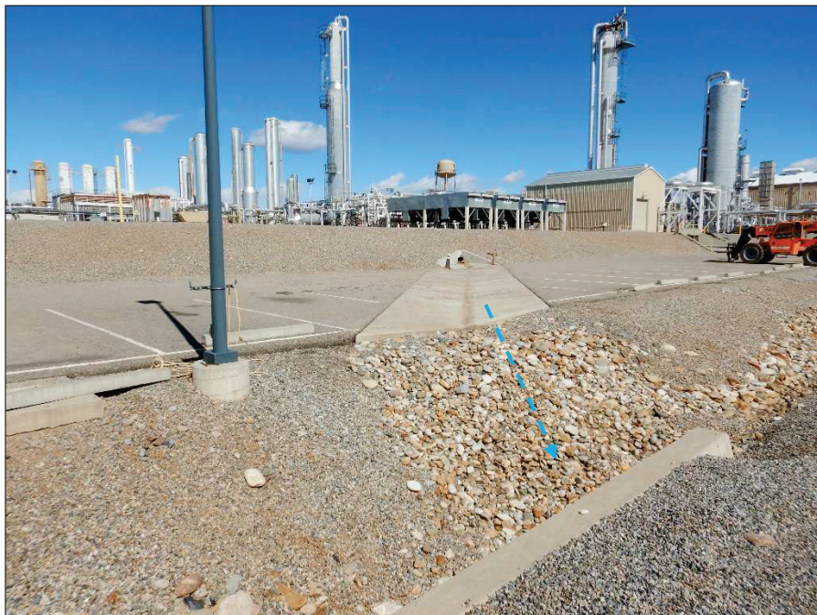
Photograph 50. View, facing Northeast, of ditch and inlet of culvert near parking lot connecting to the ditch leading to North Evaporation Stormwater Holding Pond.
