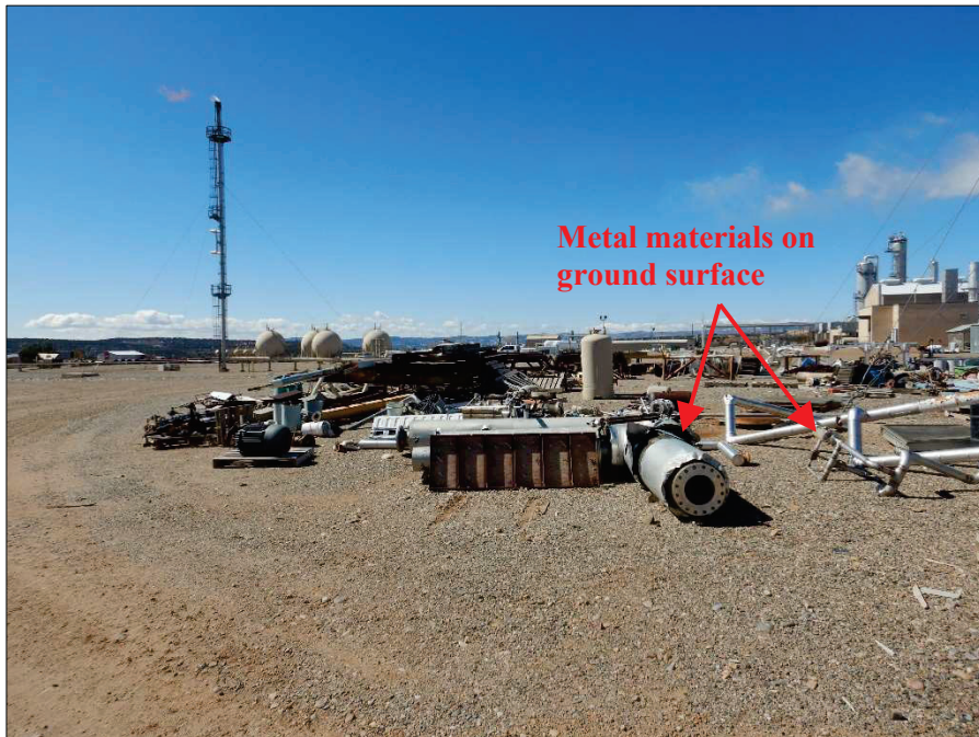
Photograph 30. Additional view, facing Southwest, of boneyard, as referenced in Photographs 28 and 29. Note materials are uncovered and sitting on the ground.
