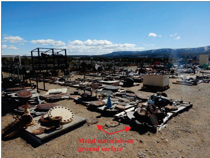
Photograph 28. View, facing Southeast, of boneyard. Note materials are uncovered and sitting on ground.
