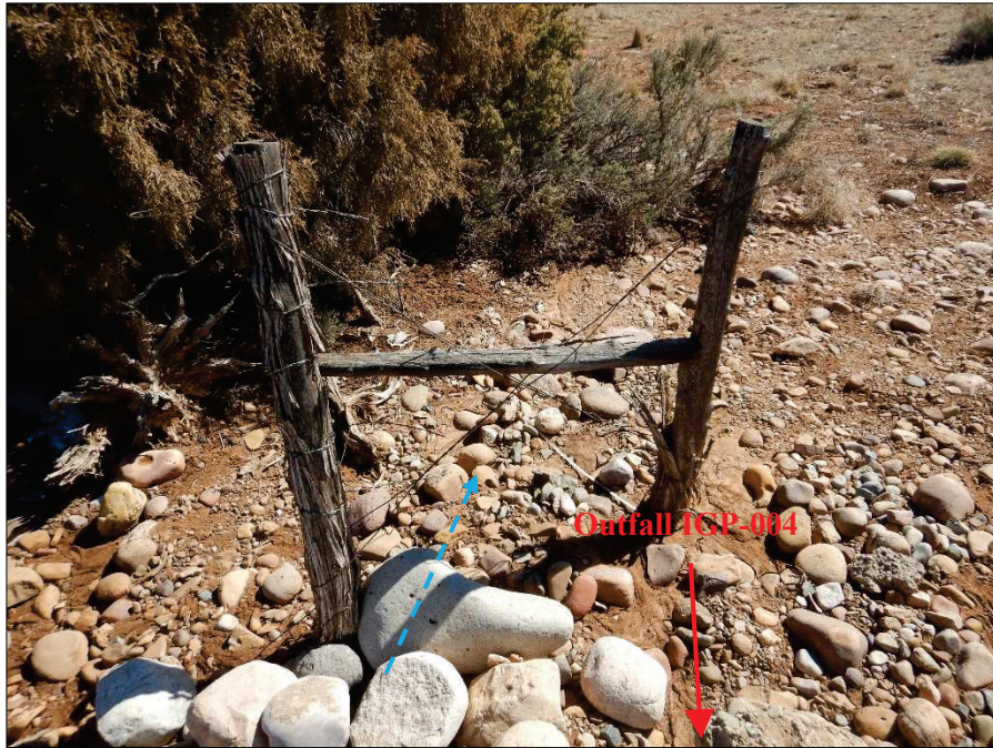
Photograph 89. Additional view, facing East, outside the fence line of Outfall IGP-004, as referenced in Photograph 88.
