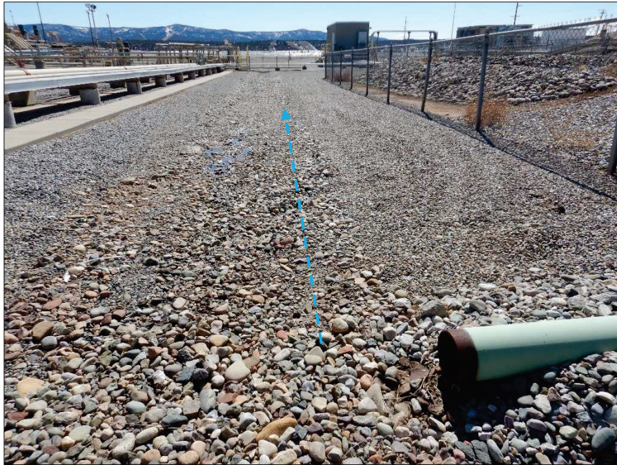
Photograph 59. View, facing South, of culvert and ditch leading from the stormwater holding pond shown in Photograph 58 towards North Evaporation Stormwater Holding Pond.
