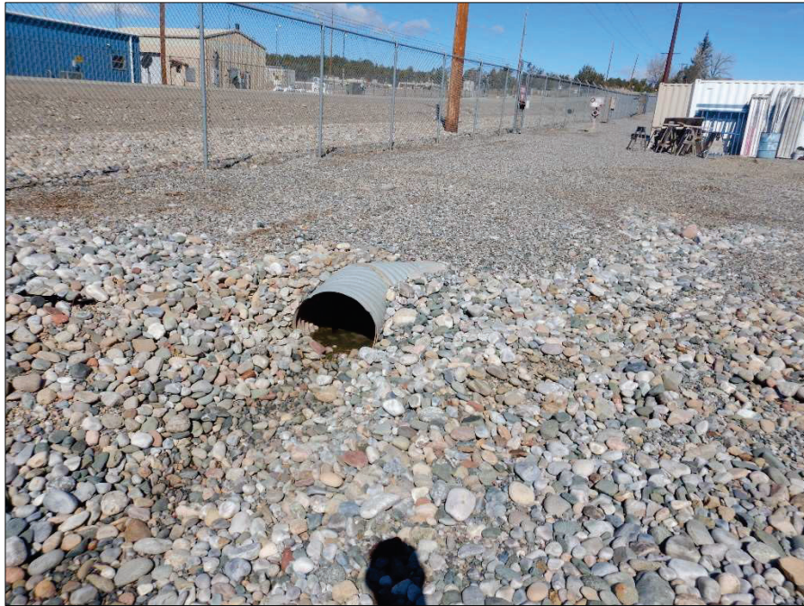
Photograph 63. View, facing North, of the outlet of a culvert connecting to Gosney Pond.
