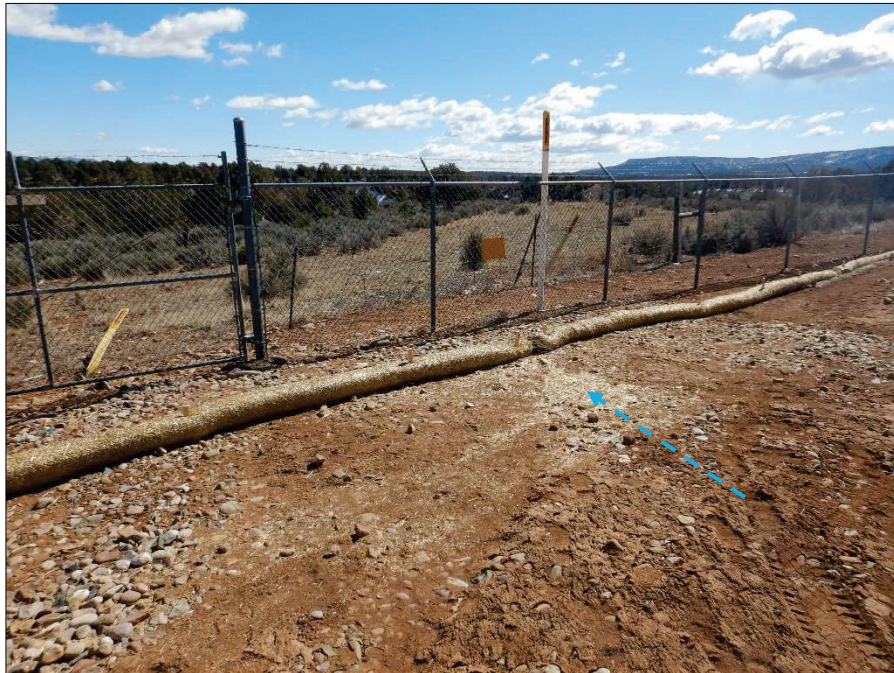
Photograph 108. Additional view, facing Southeast, of new straw wattles near Outfall IGP-004, as referenced in Photograph 107.
