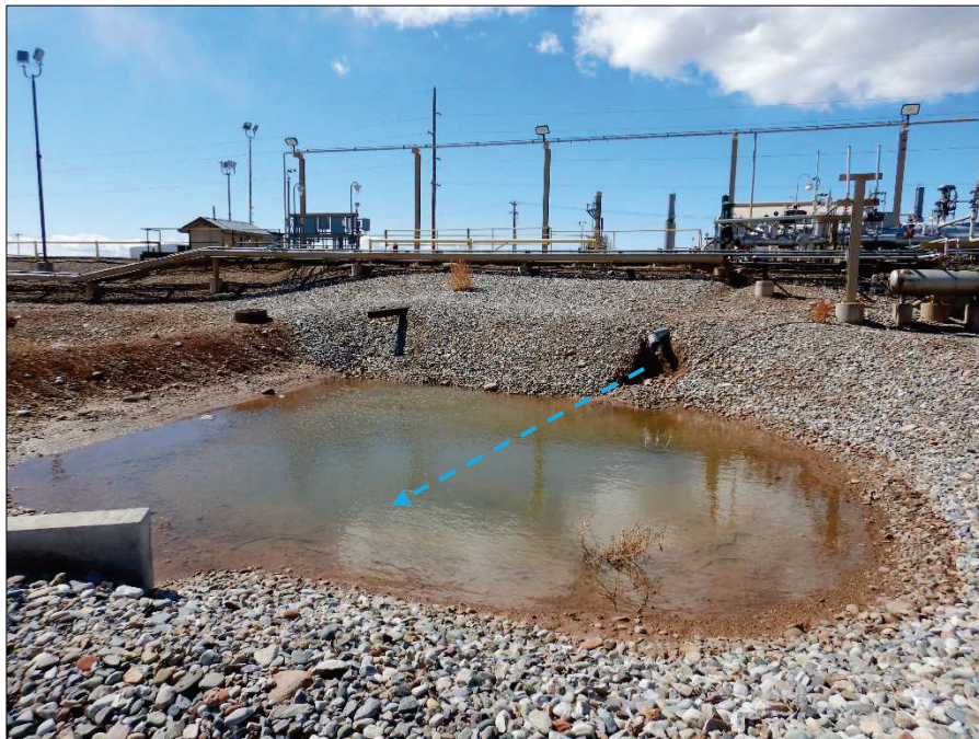
Photograph 58. View, facing West, of a stormwater holding pond that receives drainage from Drainage Area 7 and drains to North Evaporation Holding Pond. Note sediment accumulation in the pond.
