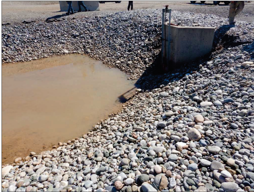
Photograph 65. Close-up view, facing Southeast, of Gosney Pond including outlet structure, as referenced in Photograph 64.
