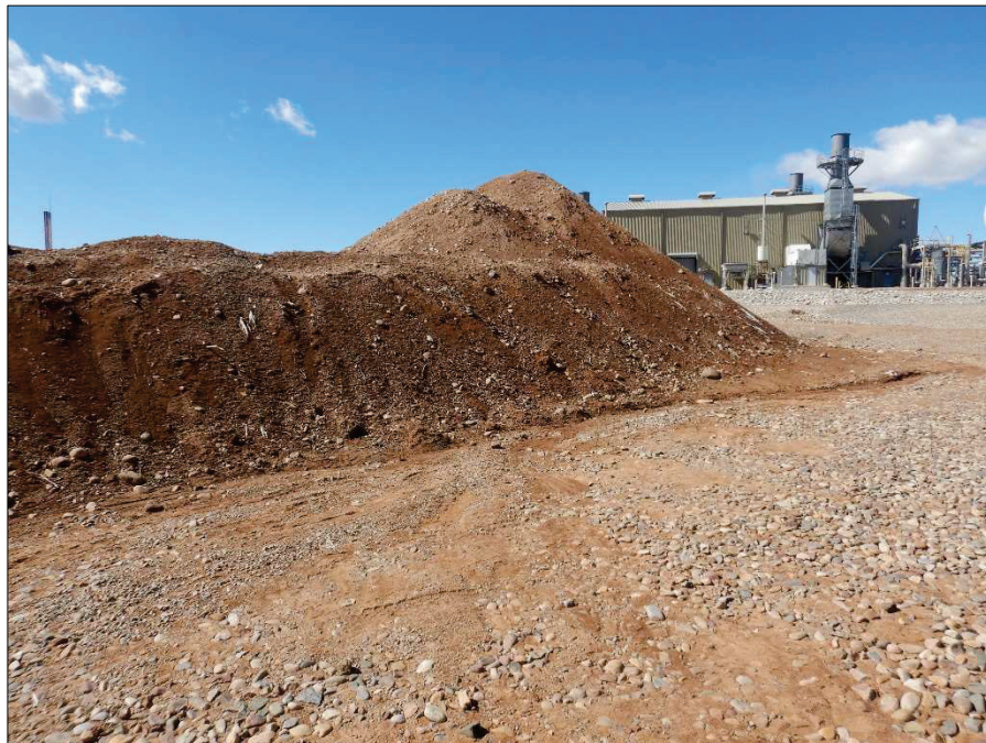
Photograph 26. View, facing Southwest, of dredged material stored in Drainage Area 15, upgradient from Outfall IGP-004. Note piles are uncovered and uncontained.
