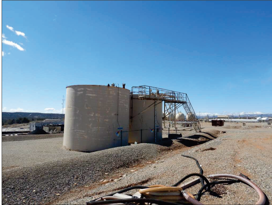
Photograph 5. View, facing Southwest, of above ground storage tanks containing industrial wastewater.
