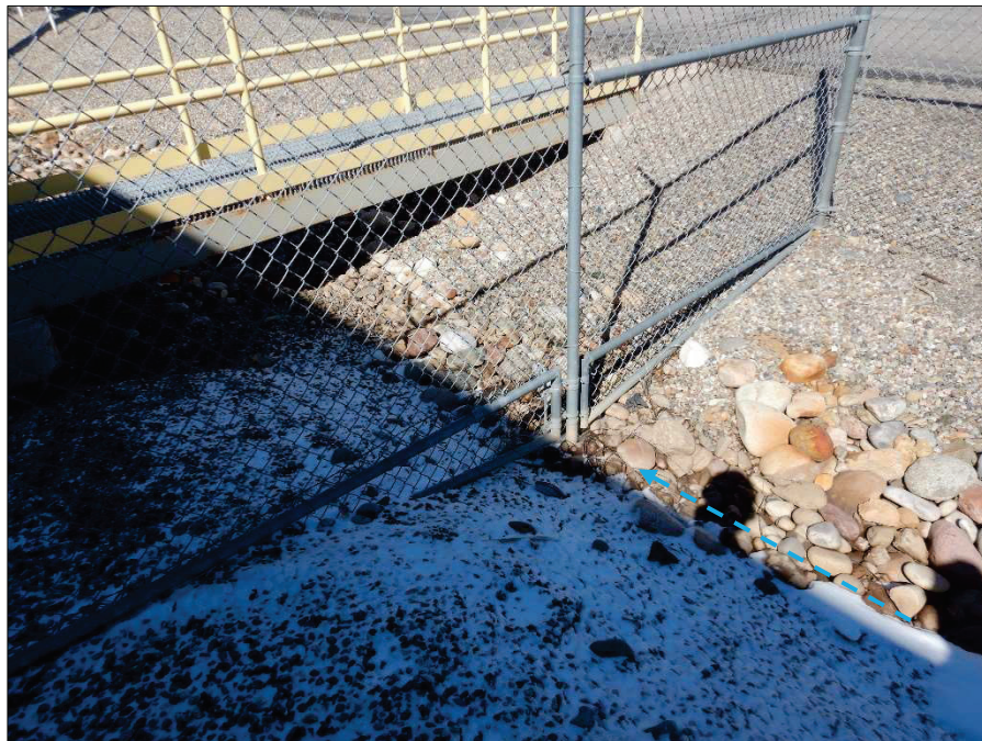
Photograph 8. Close-up view of Outfall IGP-012, as shown in Photograph 7.
