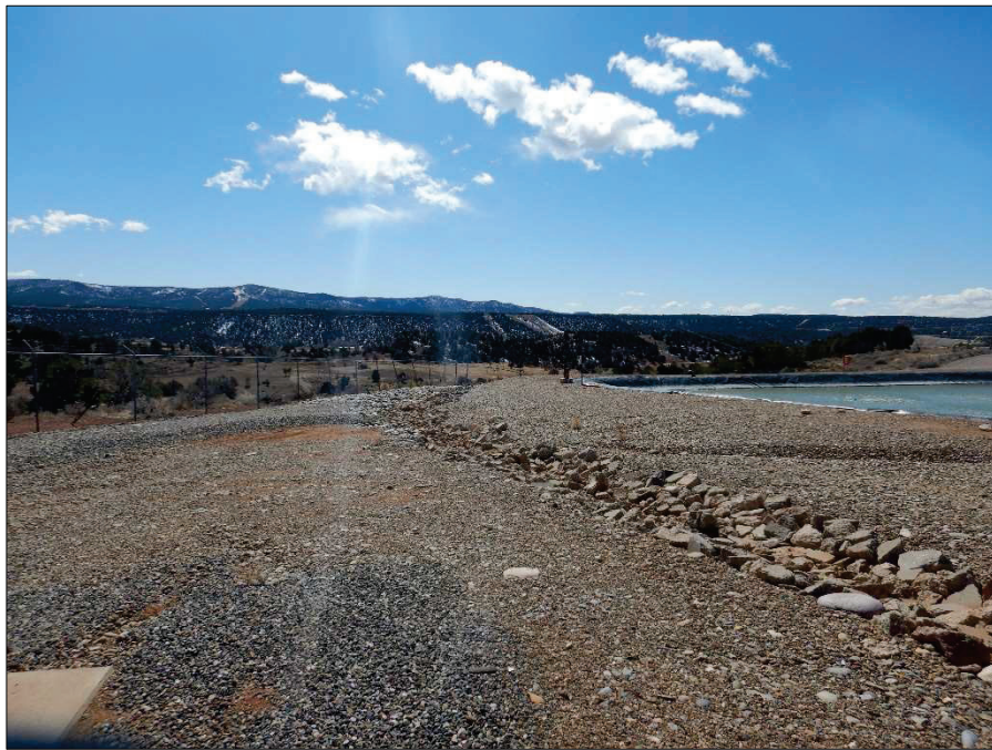
Photograph 96. View, facing South, of a ditch near East Excess Pond which drains to Outfall IGP-009, downstream from the culvert shown in Photograph 95.
