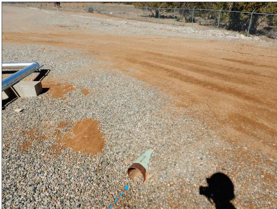
Photograph 84. View, facing Northwest, of the inlet to culvert in Drainage Area 15, which ultimately drains to Outfall IGP-003. Note accumulated sediment and gravel at the mouth of the pipe.
