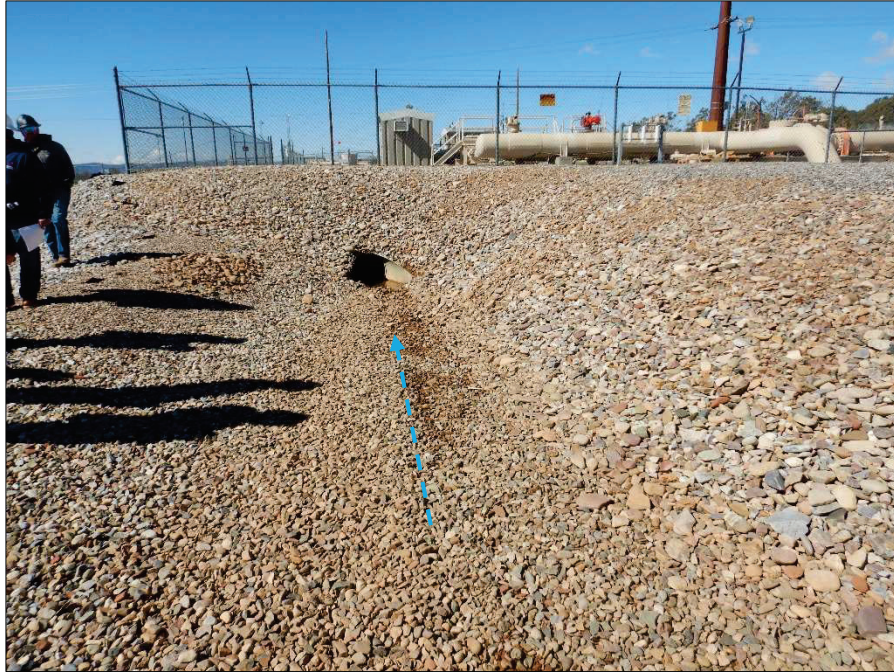
Photograph 71. View, facing West, of inlet of culvert in Drainage Area 1 leading to Outfall IGP-001.
