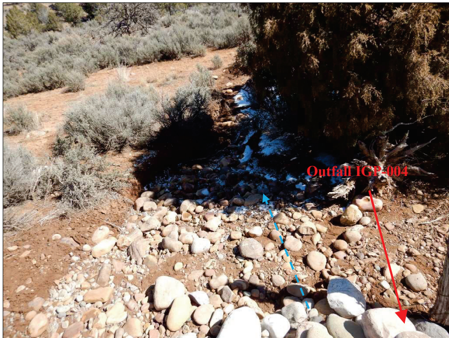
Photograph 90. Additional view, facing East, outside of the fence line of Outfall IGP-004, as referenced in Photograph 88 and 89.
