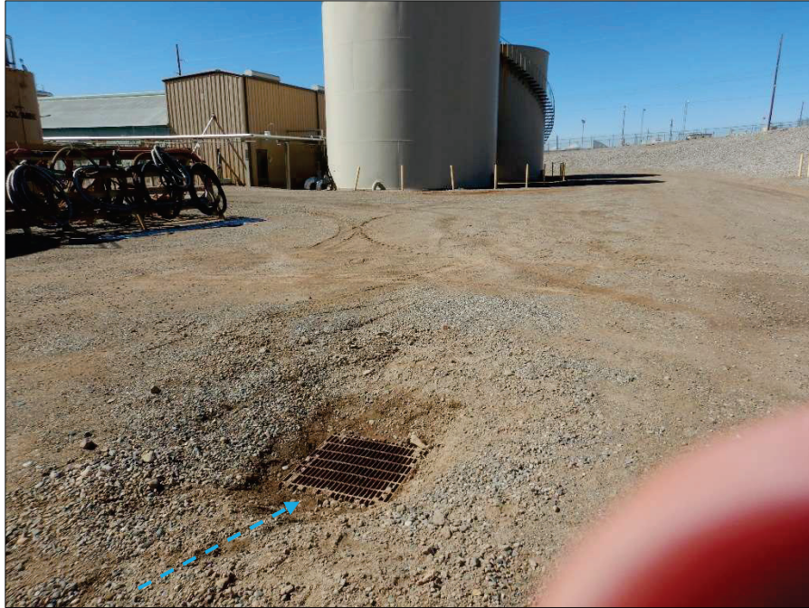
Photograph 77. View, facing West, of an unprotected catch basin in Drainage Area 2. Note loose gravel and sediment near entrance of catch basin.
