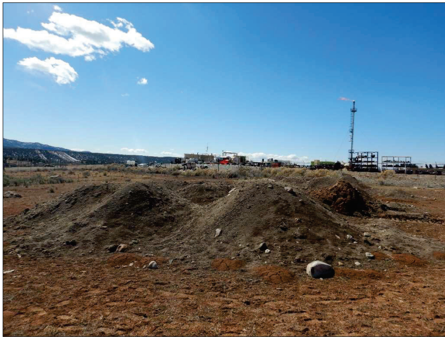
Photograph 10. Additional view, facing West, of dredged material outside of the fence line Drainage Area 15, as referenced in Photograph 9. Note piles are uncovered and uncontained.
