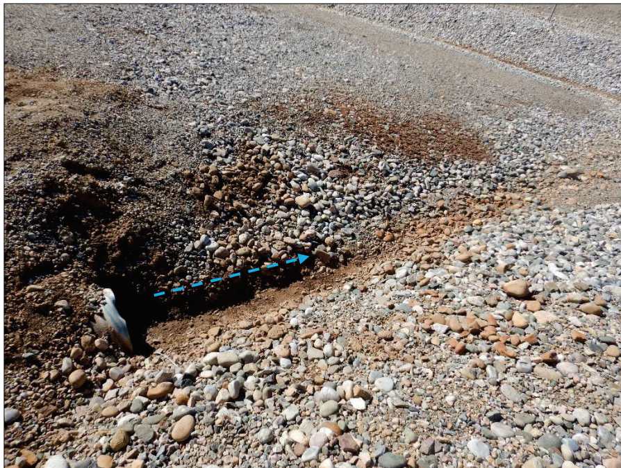
Photograph 62. View, facing Southwest, of the outlet of the culvert connecting Drainage Area 1 to Gosney Pond, as referenced in Photographs 60 and 61.
