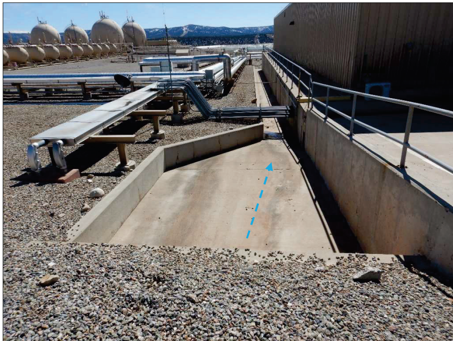
Photograph 52. Additional view, facing South, of a stormwater drainage channel connecting the locations shown in Photographs 48 through 51 to North Evaporation Stormwater Holding Pond.
