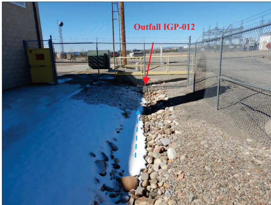
Photograph 7. View, facing North, of Outfall IGP-012.
