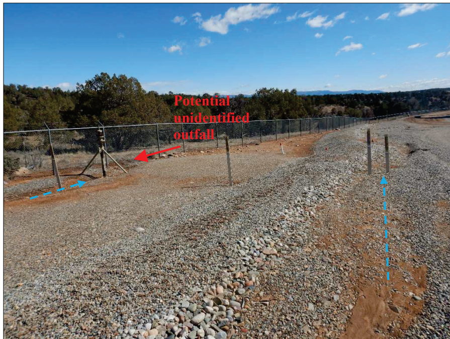
Photograph 14. Additional view, facing Northwest, of potential unidentified outfall in Drainage Area 15, as referenced in Photographs 12 and 13.
