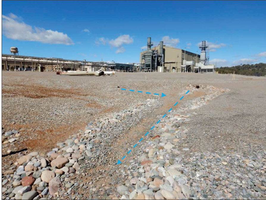
Photograph 91. View, facing Northwest, of a drainage ditch leading to Outfall IGP-006.
