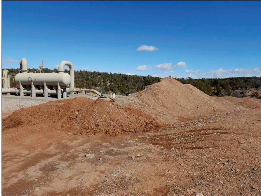
Photograph 27. Additional view, facing Northeast, of dredged material stored in Drainage Area 15, as referenced in Photograph 26. Note piles are uncovered and uncontained.
