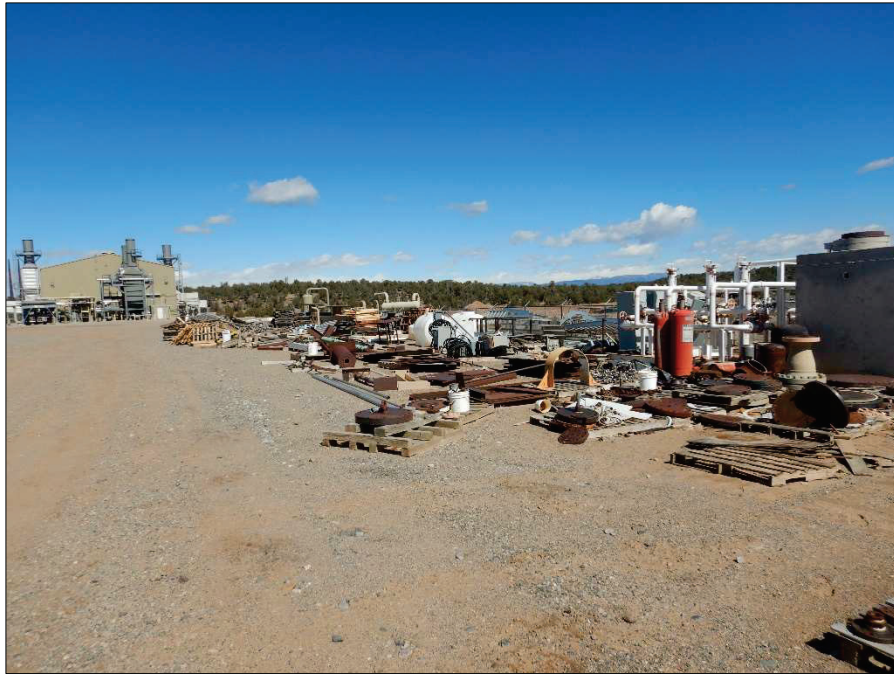
Photograph 29. Additional view, facing Northeast, of boneyard, as referenced in Photograph 28. Note materials are uncovered and sitting on the ground.
