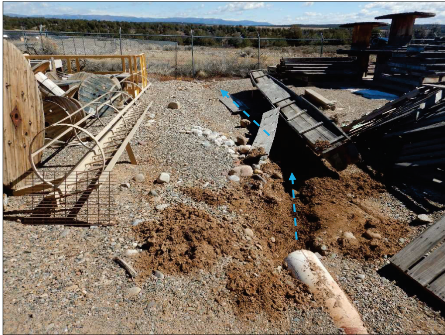
Photograph 15. View, facing East, of a stormwater drainage pathway leading from the Facility's boneyard toward the potential unidentified outfall shown in Photograph 25.
