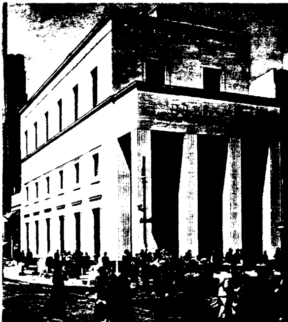
The uptown branch of the Dry Dock Savings Institution, New York City. Louis Weeks and Cross and Cross, architects. "Weathercaps" have been used extensively recently on this building, applied under the direction of the Universal Insurance Co., New York City. Other applications of lead on this building were described in LEAD, July, 1937.
