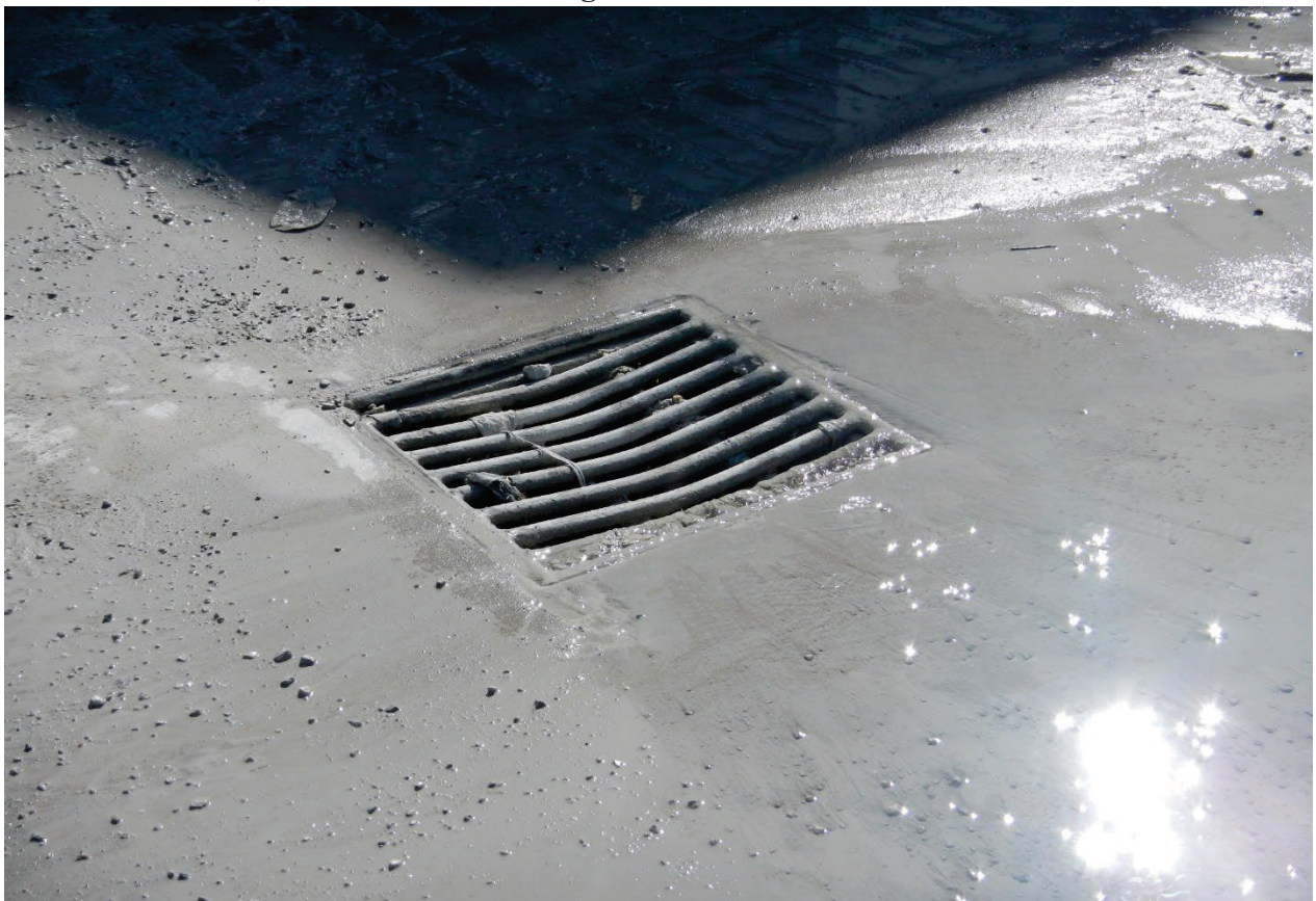
Photo 11, Process water entering a stormwater inlet that leads to Outfall 01.
