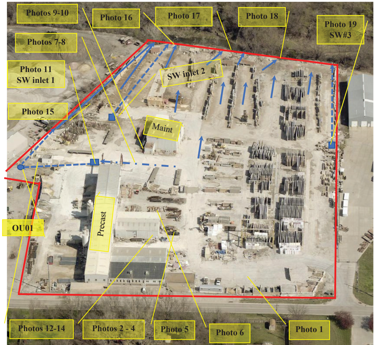
Figure 1, Enterprise Precast Concrete, Omaha Property
