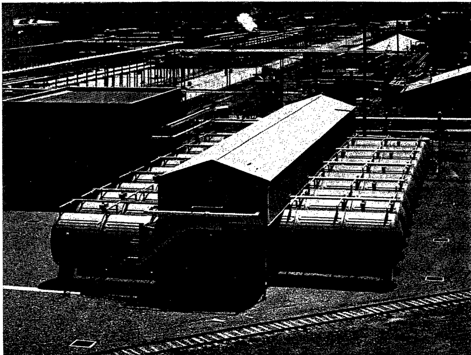
Sodium-storage facilities. Molten sodium is moved by vacuum-eduction and nitrogen-displacement.
