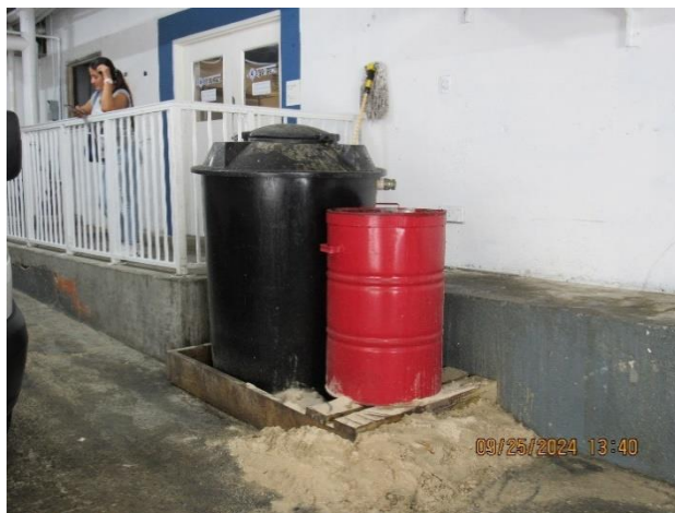
IMG 1382 -A spent cooking oil collection station in the BOH. Evidence revealed sand saturated from spent cooking oil exposed to stormwater runoff.
