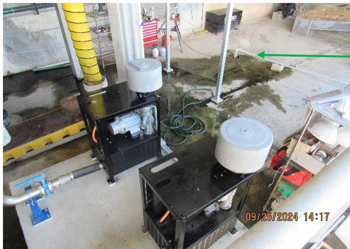
IMG 1393- Outfall B . PVC pipeline through which algae-laden water from floor in WWTP area is pumped into swale, that in turn drains into shoreline of nearby Pacquereau Bay.
