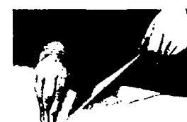
Figure 8 Use nylon sealing tool on all taped joints. This will result in a good bond and reduce air pocket and "fish-mouths." For a superior bond, use a 300F iron on the tape.
