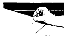
Figure 6 Cut pins to length as required and apply pre-finished fastener caps. Pins should protrude 1/8" to 1/4" above the surface of the insulation. If more than 1/4" shows, cut it off to the correct length before applying the cap. This will assure a tight fit of insulation to the surface. Apply OCF Fitting Master Tape C about the size of a pea to the inside of the fastener cap before installation to form a vapor seal.
