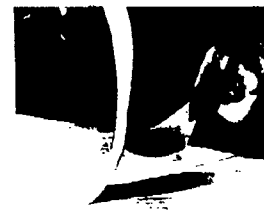
Figure 7 Apply OCF Joint Sealing Tape, Type C, to all transverse and longitudinal seams after insuring you have a dry, dust free surface. Use the nylon sealing tool to apply pressure to the joint and make a good bond. Do not remove all the release paper from the tape but rather gradually pull it back as required. This keeps dust, etc. from fouling the adhesive surface. Make sure the tape is properly aligned with the seam before it is sealed down.
