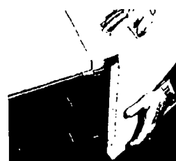
Figure 5 Install side pieces making sure the edge of the insulation is flush with the top and bottom board surfaces.
