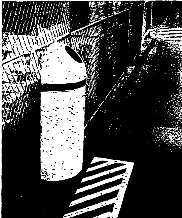
FIG 43-9— Left Rubbish disposal container made from a 55-gal drum is equipped with an automatic self-closing cover which is released in event of fire Above Waste receptacle for more-public area
