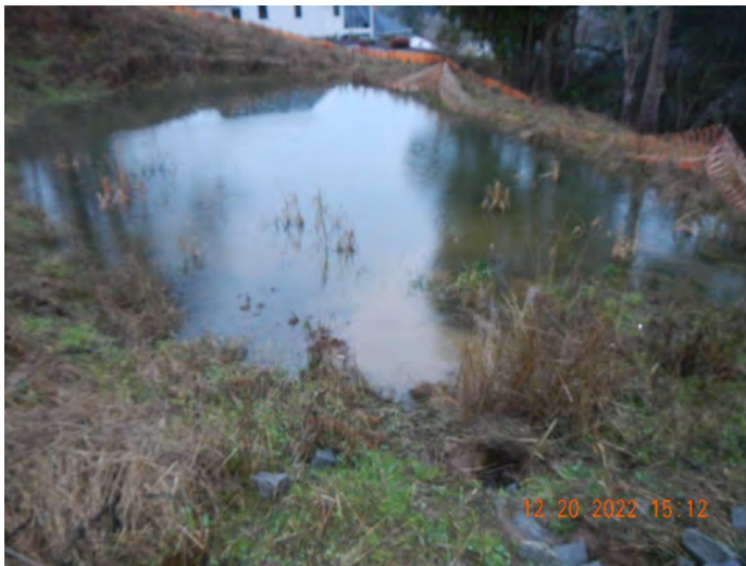
Photo #:19 (DSCN3146) Description: Facing north, photo of the inlet to the North Pond after the riprap channel.
