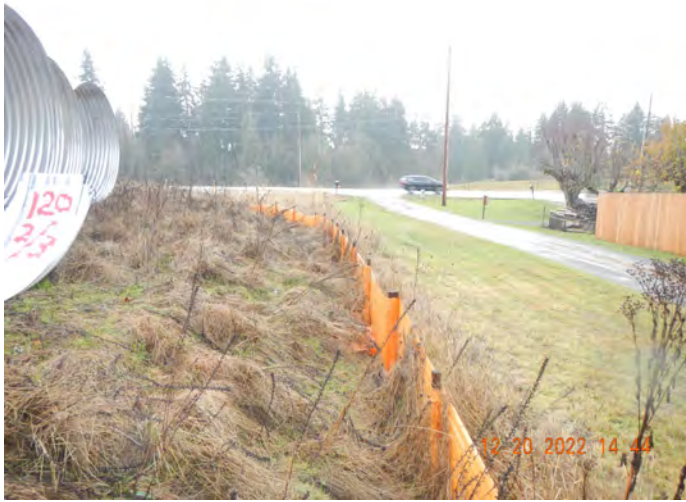
Photo #:01 (DSCN3128) Description: Facing south/southwest, photo of southwest perimeter silt fencing.
