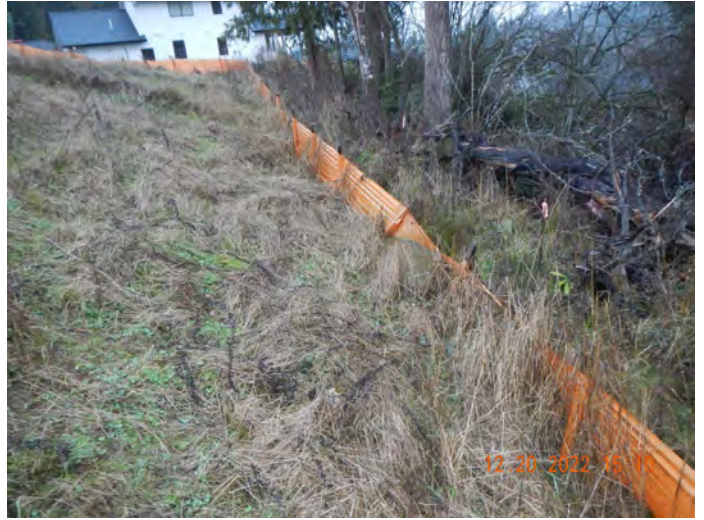
Photo #:18 (DSC3145) Description: Facing north, photo of the vegetative area east of the North Pond discharge and perimeter silt fencing.
