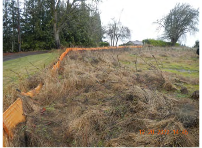
Photo #:02 (DSCN3129) Description: Facing north, photo of southwest perimeter silt fencing.
