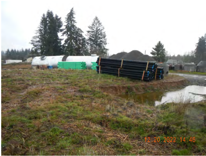
Photo #:03 (DSCN3130) Description: Facing south, photo of previous soil stockpile location and material staging area.
