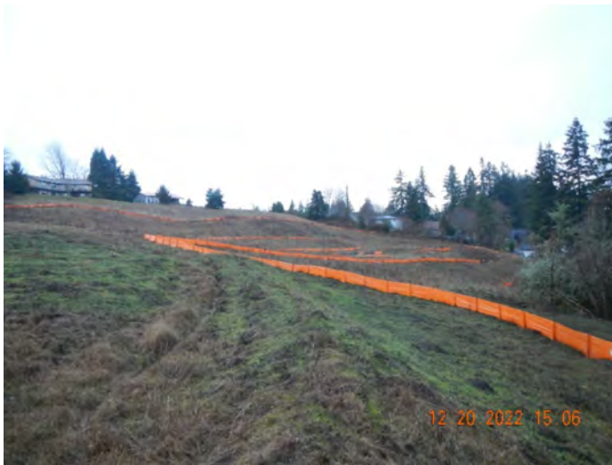
Photo #:15 (DSCN3142) Description: Facing north, photo of eastern slope and perimeter silt fencing.
