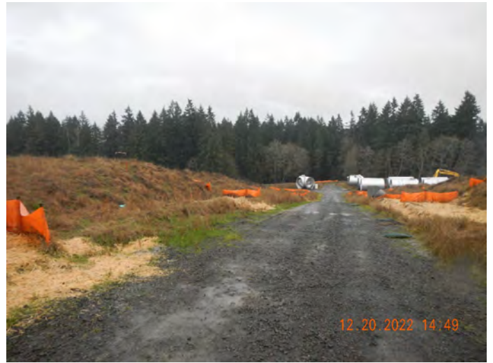
Photo #:04 (DSCN3131) Description: Facing east, photo of pond access road and BMPs.
