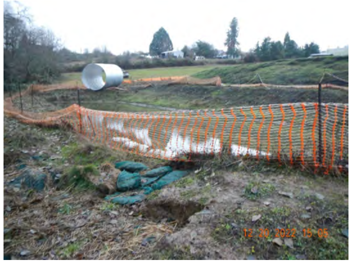
Photo #:14 (DSC3141) Description: Facing south, photo of South Pond discharge location.
