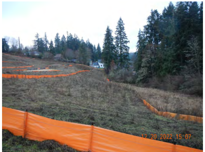
Photo #:16 (DSCN3143) Description: Facing north, photo of eastern slope and perimeter silt fencing.
