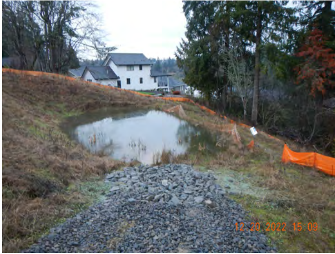
Photo #:17 (DSCN3144) Description: Facing north, photo of North Pond and riprap channel.
