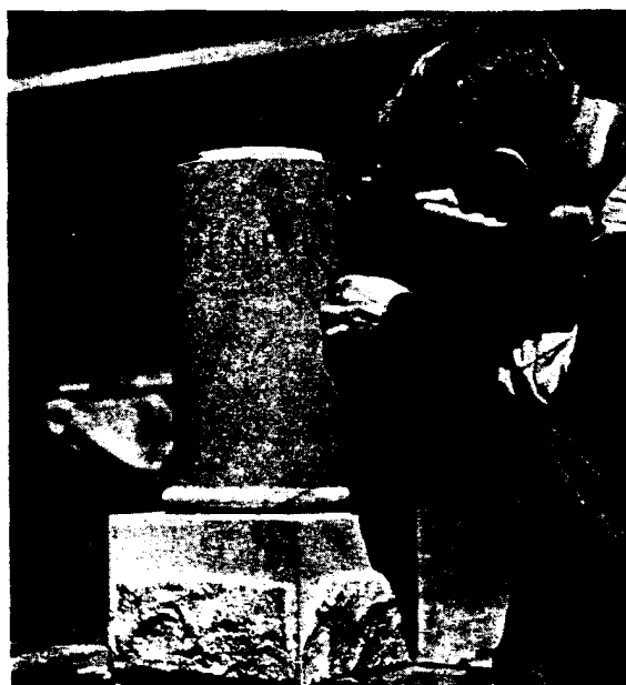
Application of lead strip in making letters on monuments.
