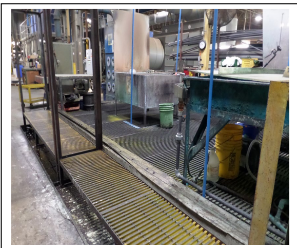
Hager. Oxidizing Line. The inspectors observed the 100-gallon capacity selenium process tank in this area. Photograph 7 taken at 10:42 a.m.
