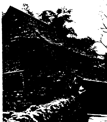
The Cotswold home and one of the lead gutters, in service for over 300 years and still in excellent condition
