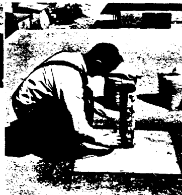
Details of sheet lead roof drain and vent pipe flashing and of a branch lead bath waste with lead vent connections wiped in for the U.S.H.A. project in Syracuse
