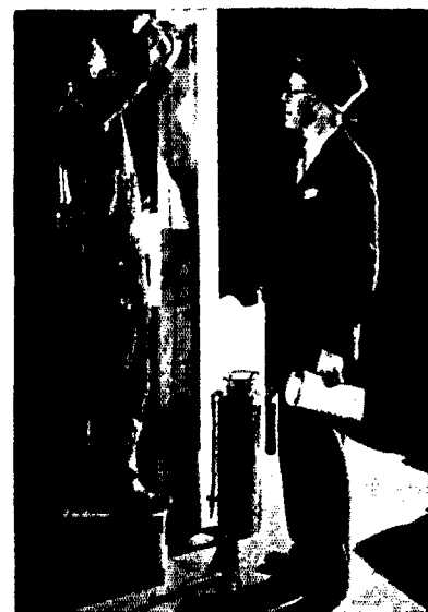
After the right type and size of extinguisher has been determined, the next step is to supervise the installation to make sure that the devices are correctly placed.
