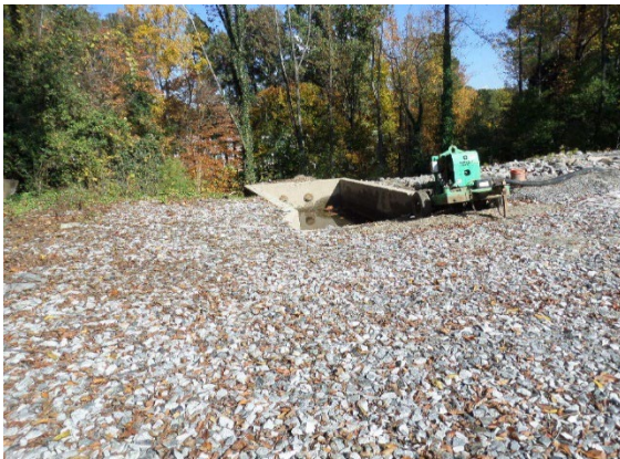
Figure 47: HTL. NWOKP. View of Northwest corner adjacent to ASR storage area. 11:42 am. View North.
