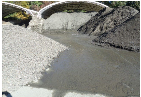
Figure 30: HTL. Bunkers. Observed stream of wastewater flowing down gradient towards Bunkers 11:18 am. View North.
