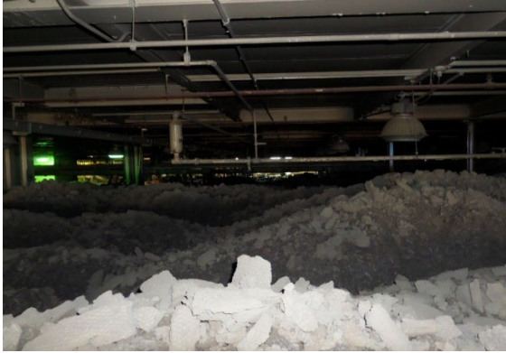
Figure 61: HTL. Old Keebler Plant (OKP). Observed asymmetrical oval shaped filter cake pile (Pile) in center area of building. 3:18 pm.
