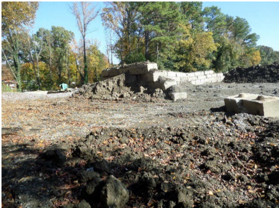
Figure 45: HTL. NWOKP. ASR storage area. Observed Mafia blocks. 11:41 am. View West.
