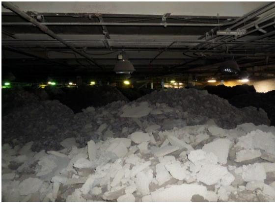
Figure 63: HTL. OKP. Pile stored in Pile from column A5 to A15 and I5 to I15 3:18 pm.
