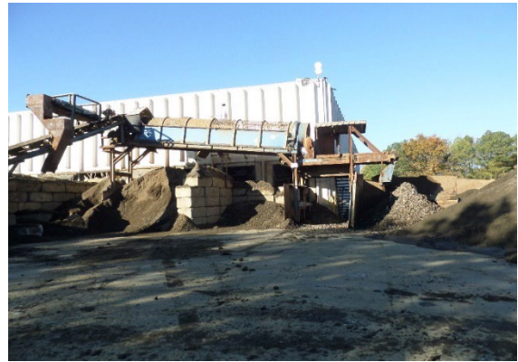
Figure 6: HTL. Old Keebler Plant. ASR loading area for TAV process 9:51 am. View North.
