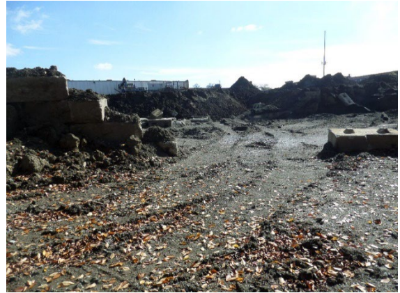
Figure 44: HTL. NWOKP. ASR storage area. Observed Mafia blocks. 11:41 am. View West
