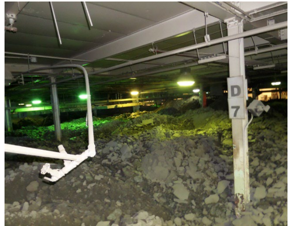
Figure 66: HTL. OKP. Observed the Pile cut to access sampling between Columns D5 to E5 3:22 pm.
