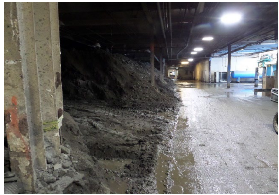
Figure 64: HTL. OKP. Observed Pile from column H5 to A5 3:18 pm.
