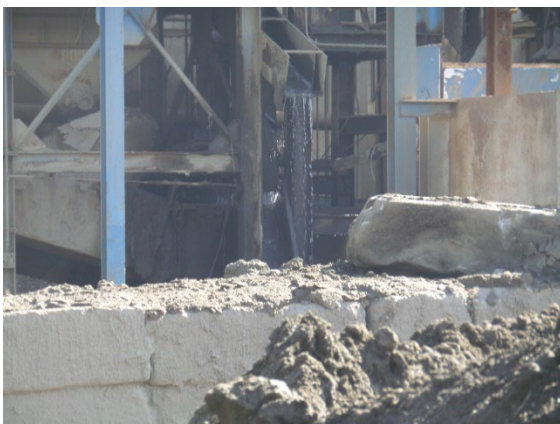
Figure 53: HTL. NWOKP. Observed release of water from process to Jig Pad Area 11:48 am. View West.
