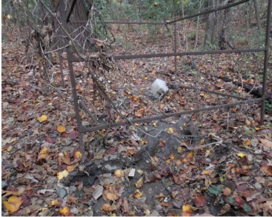
Figure 91: Access Road Area. View of woods looking down from the hill behind the Bunker drain. Observed a washed-out area from release of possible wastewater. 6:01 pm.
