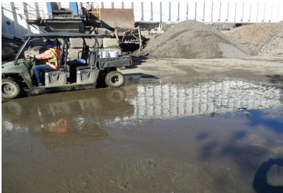
Figure 27: HTL. Adjacent Old Keebler Plant. New FVS sample containers (10) transferred for composite sampling. Observed wastewater on ground. 10:54 am.
