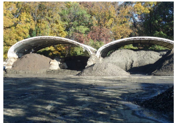
Figure 16: HTL. Adjacent Old Keebler Plant. Bunker storage. Left bunker has iron material and right bunker has 3320 Empire ASR 10:07 am. View North.
