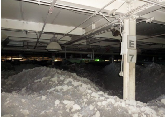
Figure 67: HTL. OKP. Observed the Pile cut to access sampling between Columns D5 to E5 3:22 pm.
