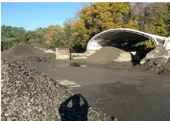
Figure 5: HTL. Observed right bunker for ASR storage. Observed sand in piles. Observed wastewater comingled. 9:49 am. View North to Northwest.
