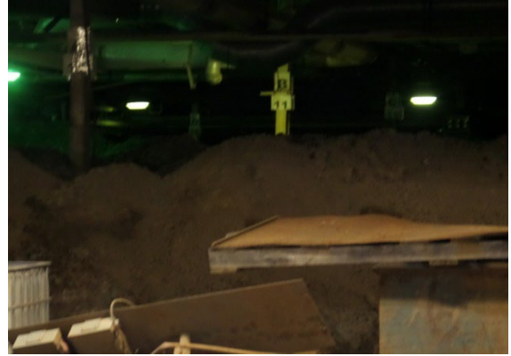
Figure 68: HTL. OKP. Observed the Pile between Columns A9 to A11 and A14 3:32 pm.
