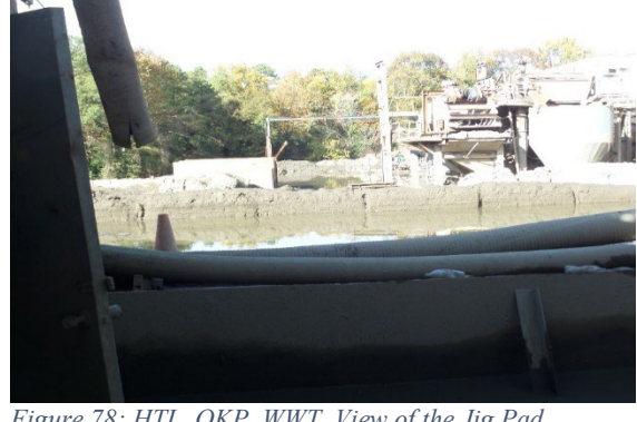
Figure 78: HTL. OKP. WWT. View of the Jig Pad. Observed Jig Pad full of wastewater possibly overflowing to the ground. 4:01 pm.
