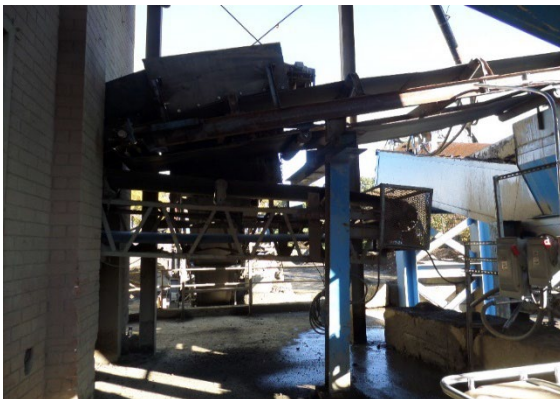
Figure 23: HTL. Adjacent Old Keebler Plant. Observed conveyor system for new FVS process. 10:29 am.
