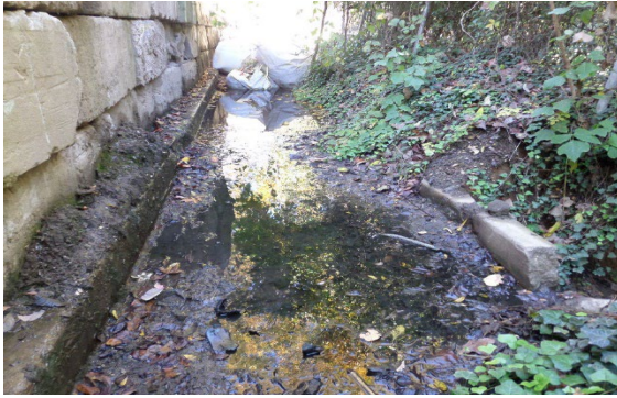
Figure 37: HTL. Bunkers. Observed concrete culvert near drain had water behind Bunkers. Observed drains to outfall downhill to woods near Access Road Area. 11:27 am.
