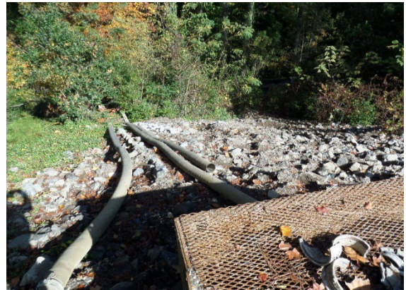
Figure 48: HTL. NWOKP. View of Northwest corner adjacent to ASR storage area. Down gradient of hill toward stormwater outfall. 11:44 am. View North.
