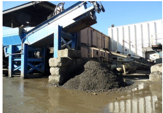
Figure 28: HTL. Adjacent Old Keebler Plant. Continue to generate New FVS heavies from back end. Process feed stopped. Observed wastewater on ground. 10:58 am.
