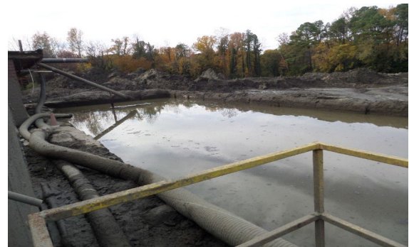
Figure 82: HTL. OKP. WWT. View of Jig Pad. Observed Jig Pad full of water adjacent to piles of possible filter cake/waste solids adjacent to ASR storage area. 4:28 pm.
