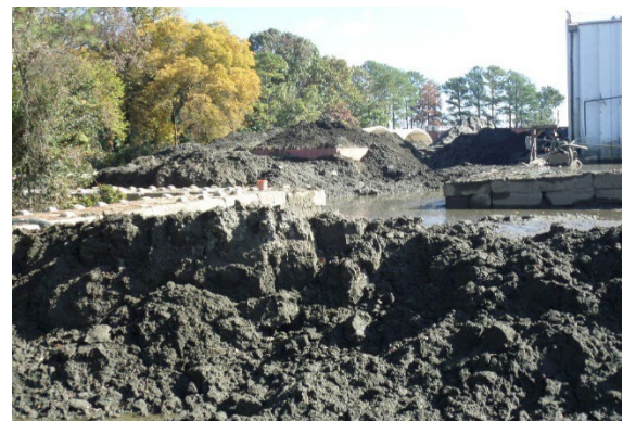
Figure 54: HTL. NWOKP. Observed possible filter cake/waste solids in ASR storage area, Observed water in Jig Pad Area. 11:50 am. View West.
