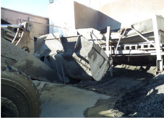
Figure 13: HTL. Adjacent Old Keebler Plant. Observed front end loader with bucket feeding ASR to process. 10:02 am. View toward building.
