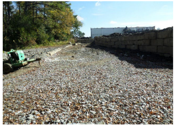
Figure 46: HTL. NWOKP. ASR storage area. Observed Mafia blocks. 11:42 am. View West.
