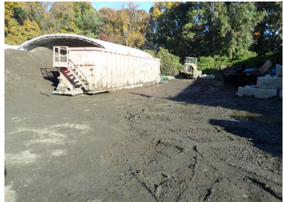
Figure 2: HTL. Observed right bunker and concrete culvert area 9:49 am. View North.
