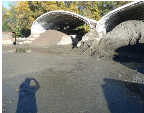
Figure 4: HTL. Observed left bunker storing possible recovered iron and right bunker for ASR storage. Observed wastewater on the ground 9:49 am. View North.
