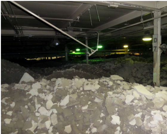
Figure 65: HTL. OKP. Observed the Pile cut to access sampling between Columns D5 to E5 3:22 pm.
