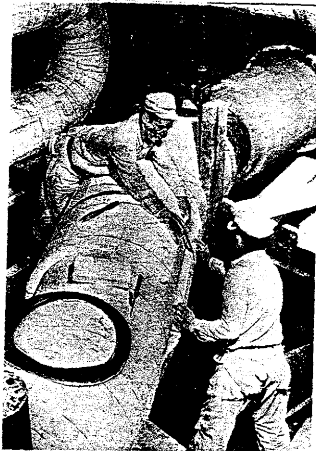
STEAM MAINS being covered with high-temperature insulation
