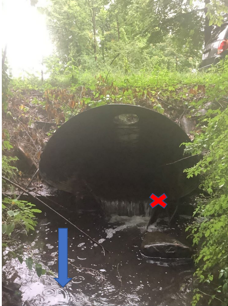
Dearborn: An in-stream sample of Bloody Brook collected at the stream culvert on Dearborn Road. Flow direction indicated by a blue arrow. Sample point indicated by a red "X".
