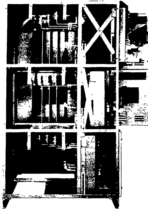
Side Plate of low voltage switchgear unit removed to show details of pantograph action for breaker withdrawal.
