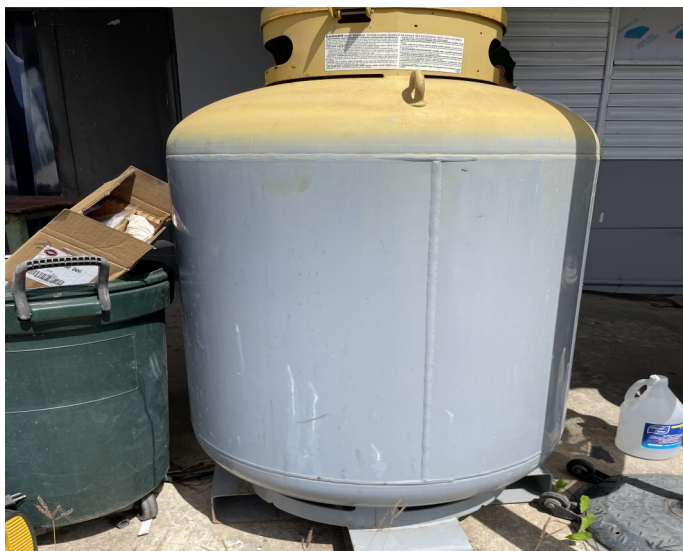
Picture 103 - UPR BUILDINGS & LAND DEPARTMENT- At the At the Refrigeration Shop, there were two (2) 1,000 pounds steel tanks with discarded refrigerants not marked with the words, "Used Refrigerant." No hazardous waste determination has been made nor recycling or reclaiming program evidenced.
