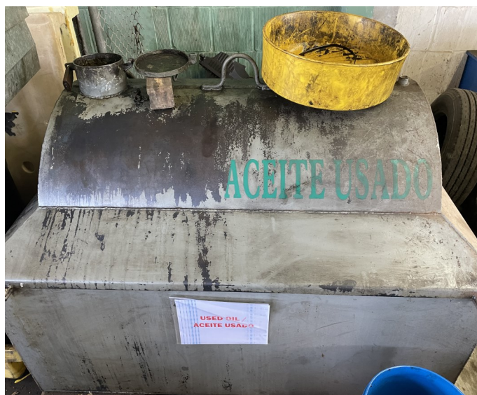
Picture 99 - UPR BUILDINGS & LAND DEPARTMENT - At the Mechanic Shop there was one (1) 200-gallon double wall Used Oil Steel Tank marked with the words, "Used Oil." However, there were old and new used oil spills and stains on the concrete floor of the used oil.
