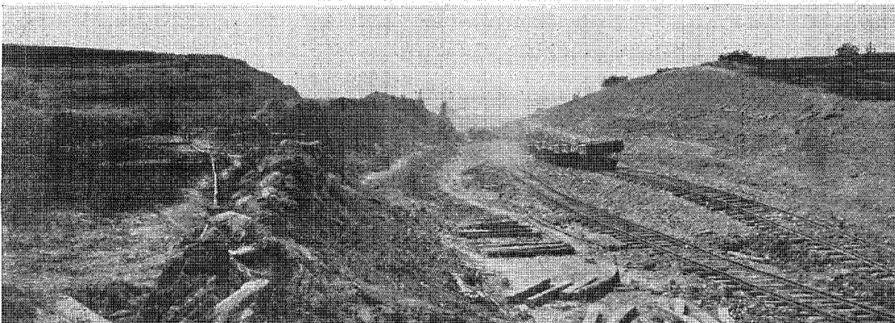
A section of the Hoffmire Cut, looking west. It is a broad, deep gash and will accommodate two tracks
