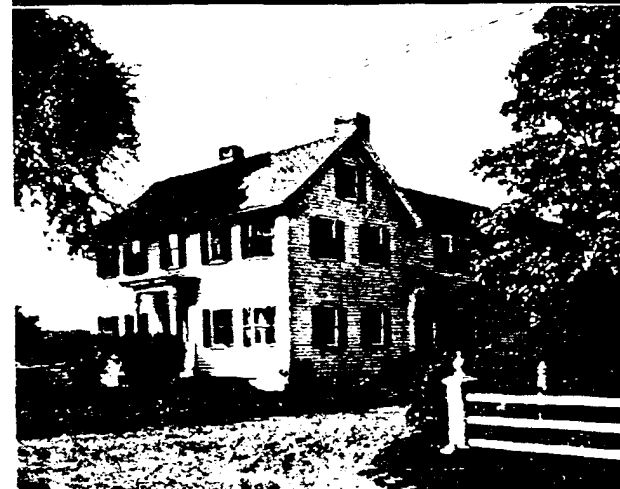
The Jesse Tapley house, built about 1830, shows little evidence of having been begun as a shoe factory. Pure white lead paint helps the attractive entrances to impart a homelike atmosphere
