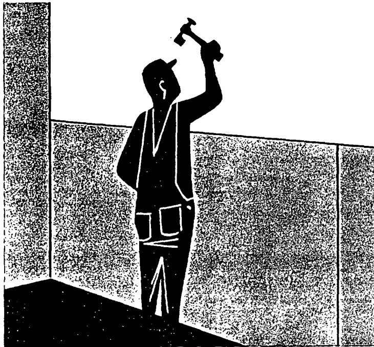
c. Next, apply face layer on upper walls and temporarily secure to the underlying framing with supports, spaced 16" to 24" c. to c. (Ceiling and sidewall end joints may occur between underlying members. In such cases, provide temporary bracing as for "Back-Blocking" ... see Figure 16—Folder WB-15.) Predecorated SHEETROCK gypsum wallboards are normally applied with the long edge parallel to the underlying members (vertically).
