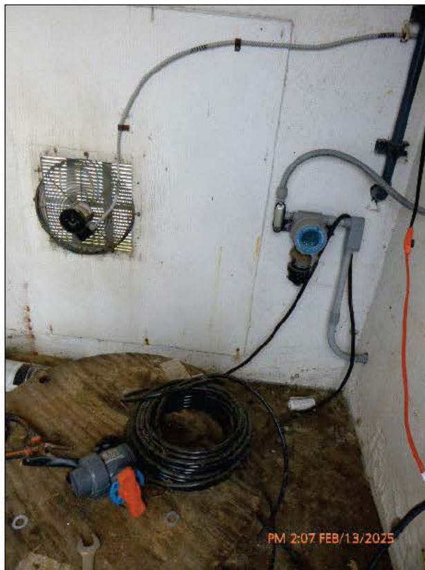
Photograph 25. 2/13/2025 2:07 pm P1010282.JPG Description: Plant #2. Chlorine gas room with ongoing repairs.
