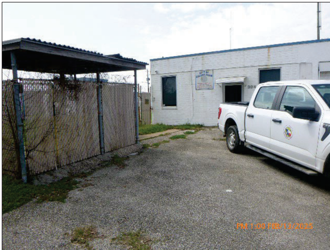
Photograph 8. 2/13/2025 1:00 pm P1010240.JPG Description: Plant #1. Office building and fence around facilities.
