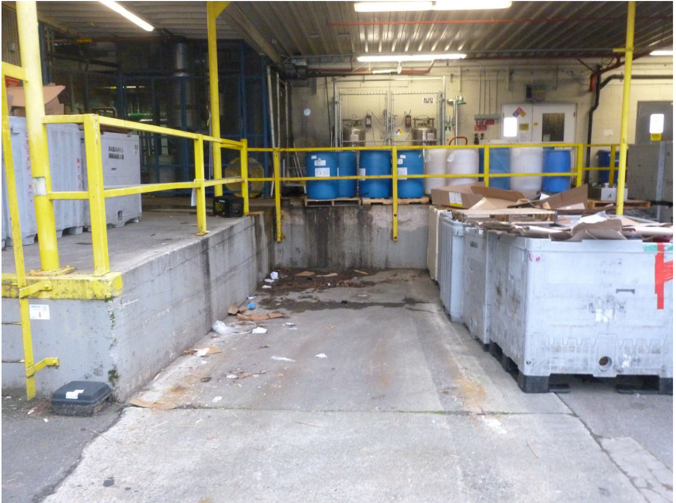
Photo 2 / P1010199 – Dock, Out of Service
