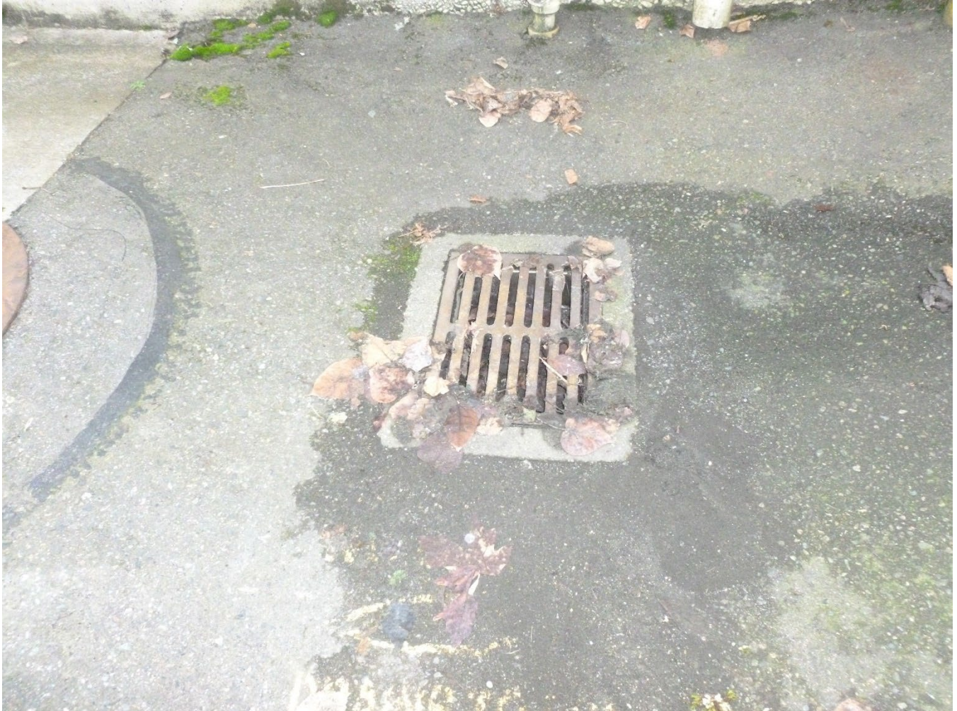
Photo 7 / P1010204 – Catch Basin, CB12
