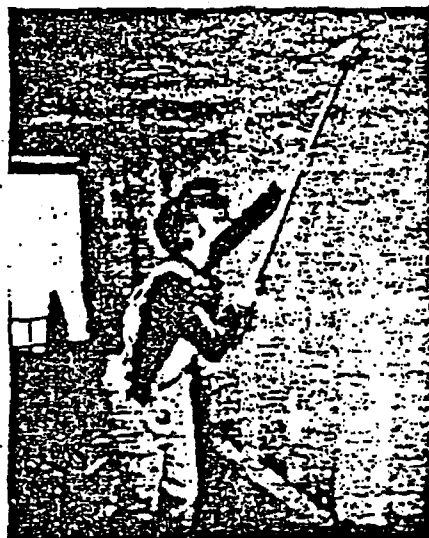
Sanding of dried spackle material with a pole sander. Dust concentrations here often exceed the current asbestos standard.
