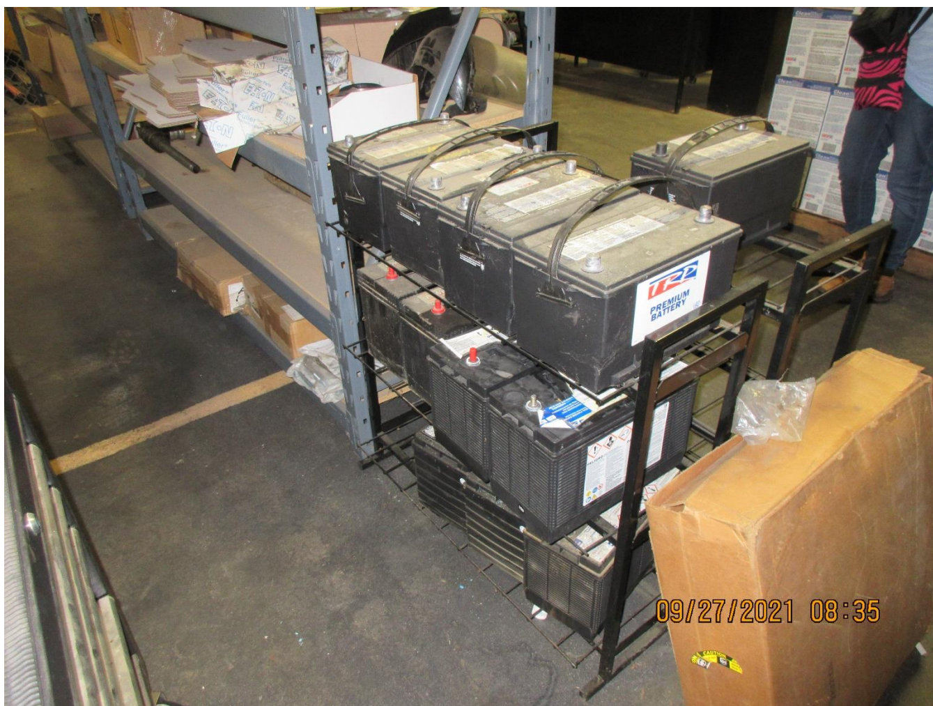
Photo 1 – Lead acid universal waste batteries in the Mechanic Shop
