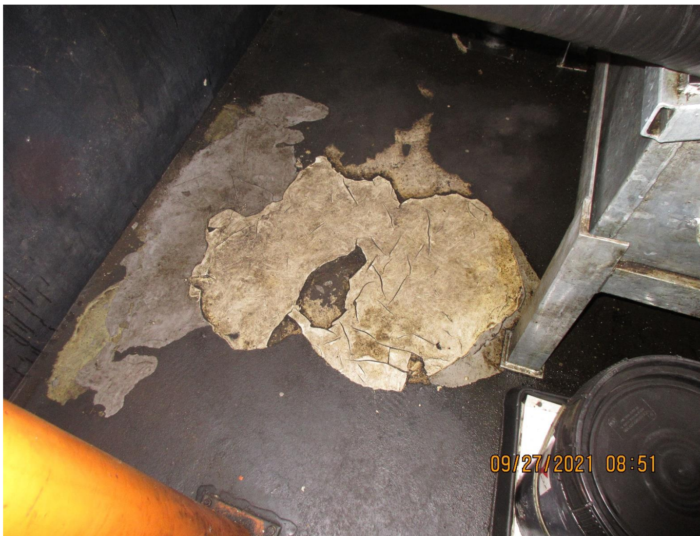
Photo 2 – Floor of secondary containment system for facility’s permitted hazardous waste storage tank.
