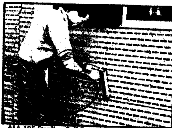
ALA-125 Stapling Self-Furred Exterior Stucco-Lath
