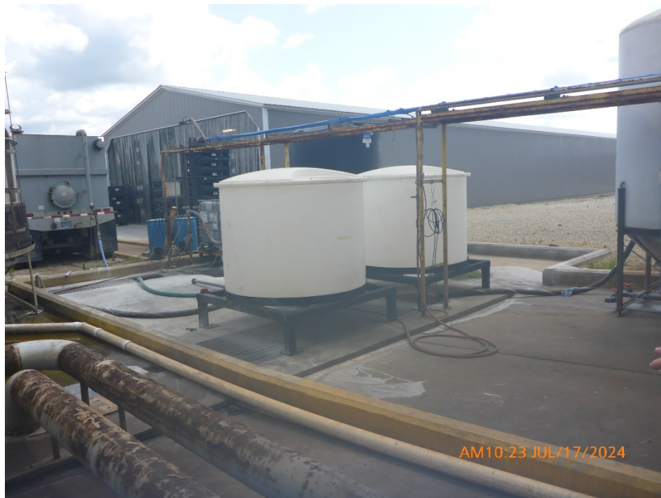
Photograph 4: View of the future wastewater pretreatment area. The wastewater holding tank is below ground and not visible.
