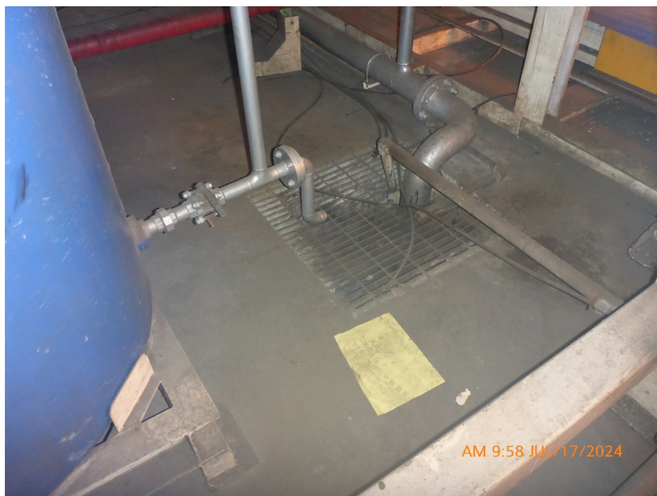
Photograph 2: Drain from the phosphate line to the wastewater pit.
