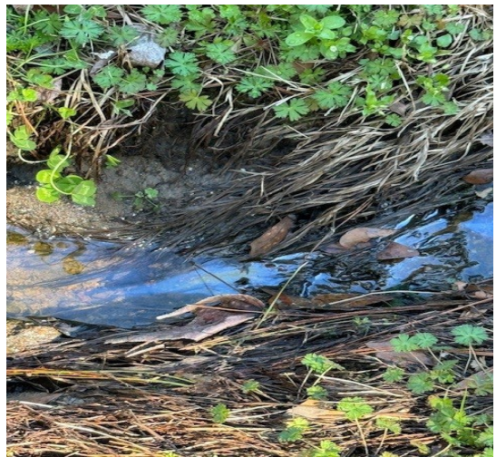
Photo-12 Oily sheen in the drainage ditch
