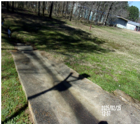
Photo-8 Concrete Stormwater Channel
