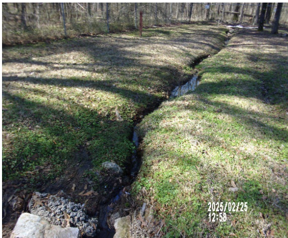
Photo-9 Drainage ditch
