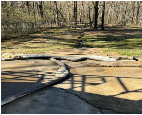
Photo-7 Spill Boom near Frac Tank
