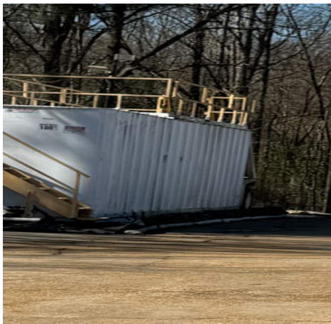
Photo-1 21,000-gallon Frac Tank
