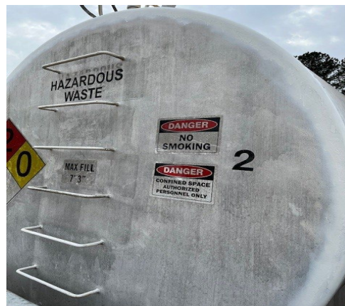
Photo-28 Tank #1 Repainted
