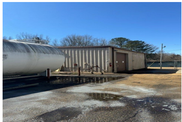
Photo-39 Absorbent Material on the gravel
