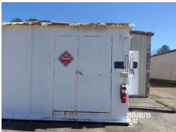
Photo-35 Container Storage Flammable Storage Shelter
