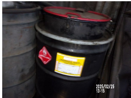
Photo-34 SAA Container (Return and Fill Station)
