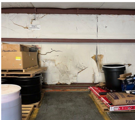
Photo-21 Insulation Repaired (Permitted Storage Area)
