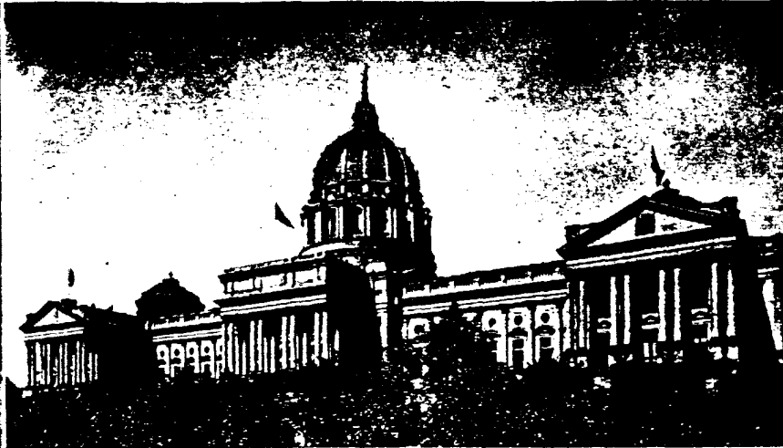
General view of Pennsylvania State Capitol Building with leadwork on dome completed.
