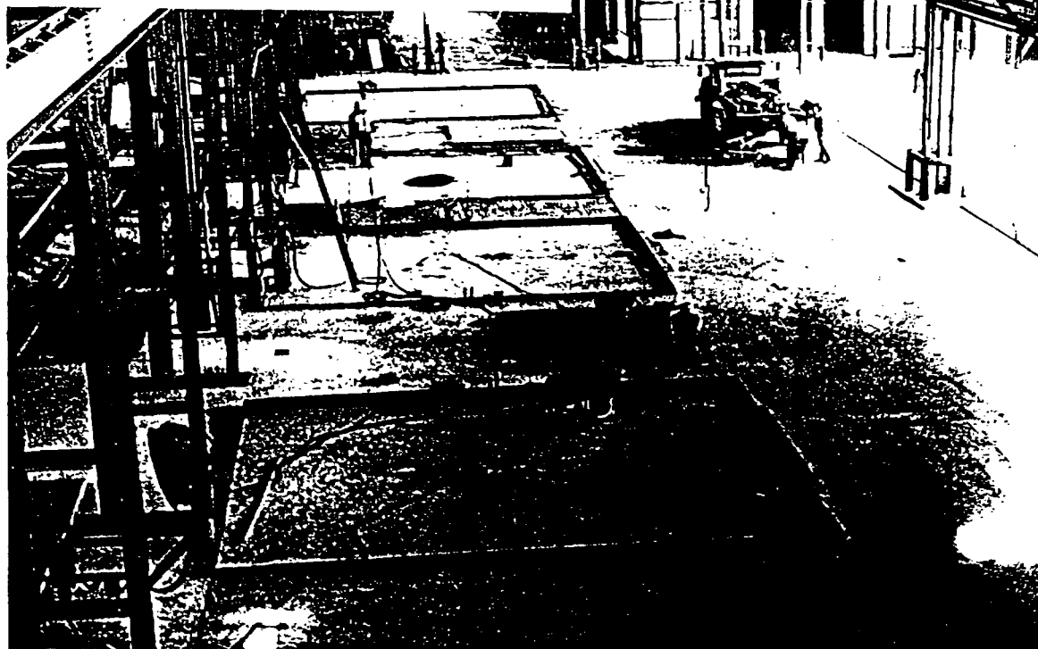
Foundations and Floor Slab, Bldg. 034 Looking South, 8-31-73
