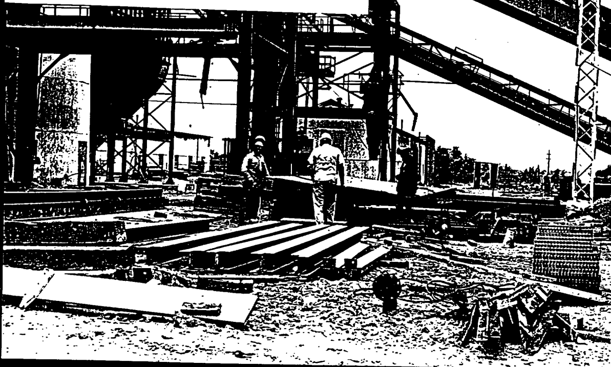
Power House Structural Steel For Electrostatic Precipitator Looking North, Auth #731109 5-15-74
