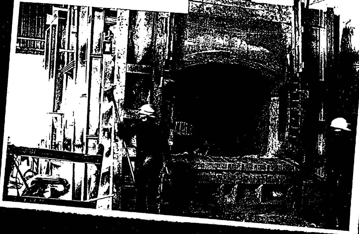
Demolition of Atomizer Furnace Looking North, 11-28-73 Auth. #720702
