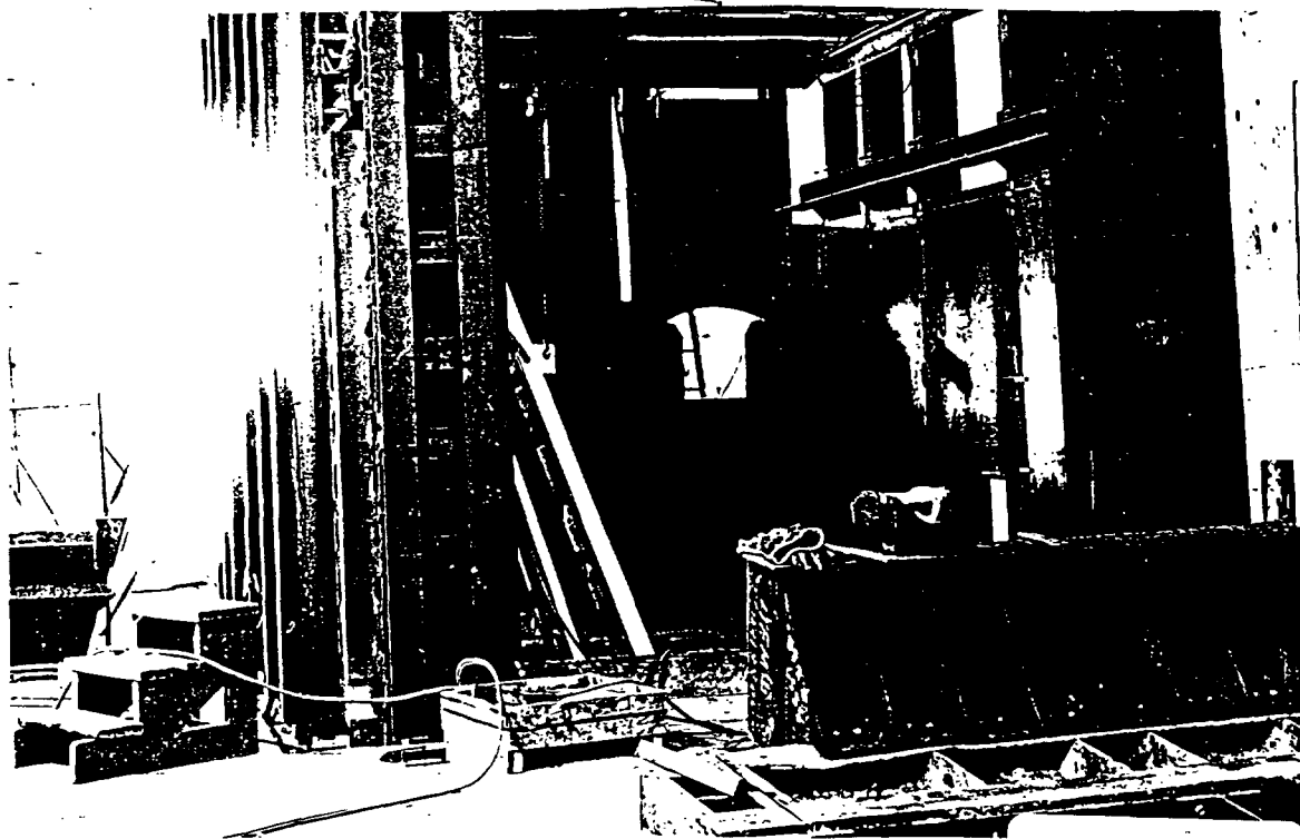
BLDG. 034 - HOLDING FURNACE #12 LOOKING EAST AUTH. RS-720769 DATED 12/20/73
