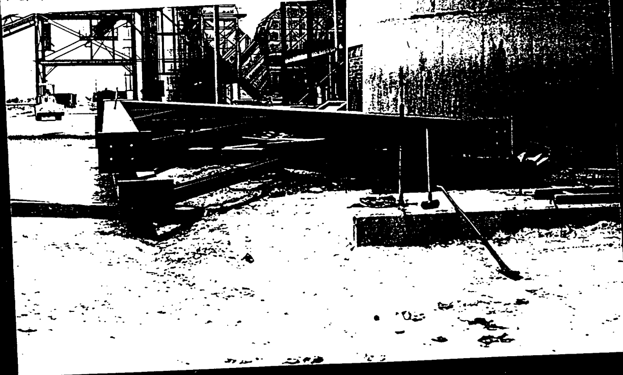
Power House Precipitator Support Columns Boiler No. 2, Auth. #731109 4-17-74
