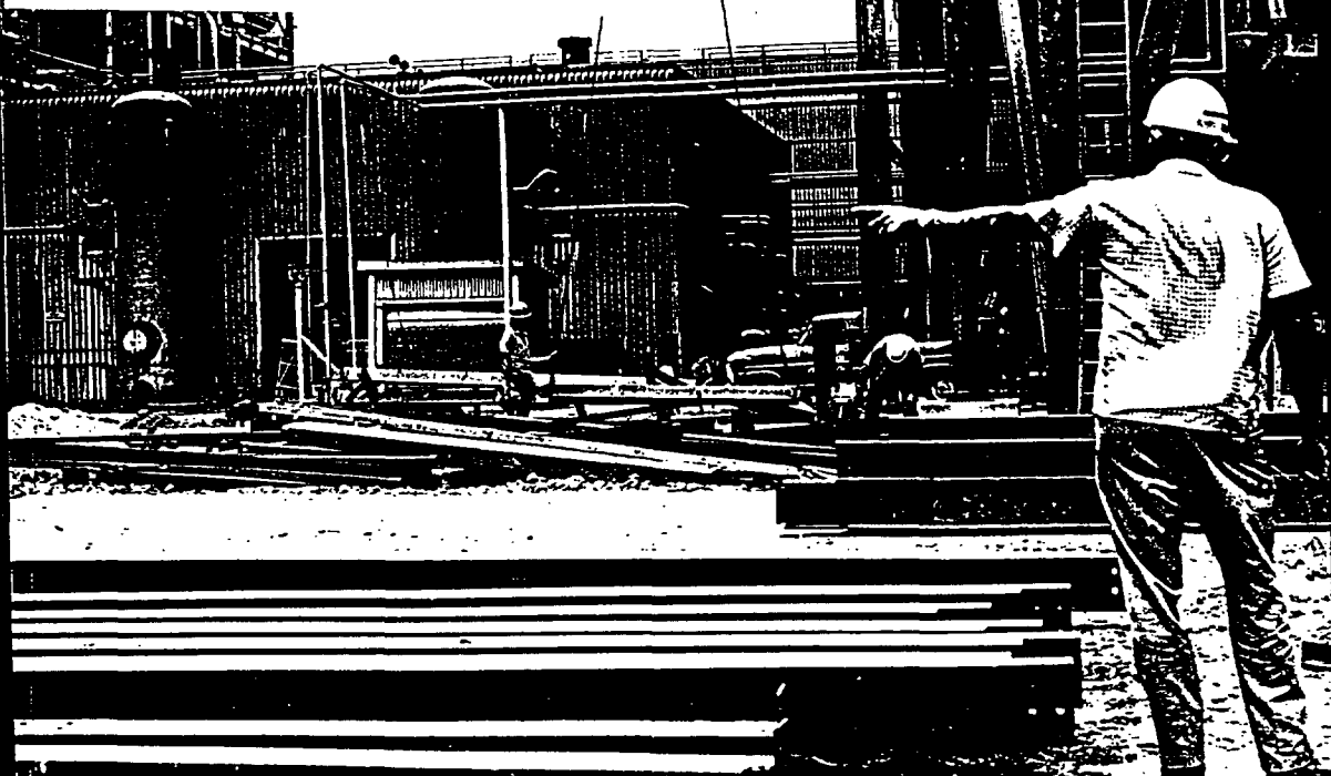
Power House Precipitator Structural Steel Looking West, Auth #731109, 5-15-74
