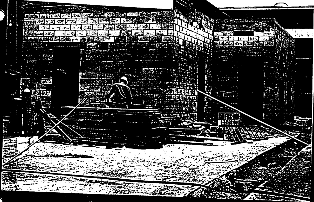
A-446 Control Building 60-D Looking South Auth #731241, 5-15-74
