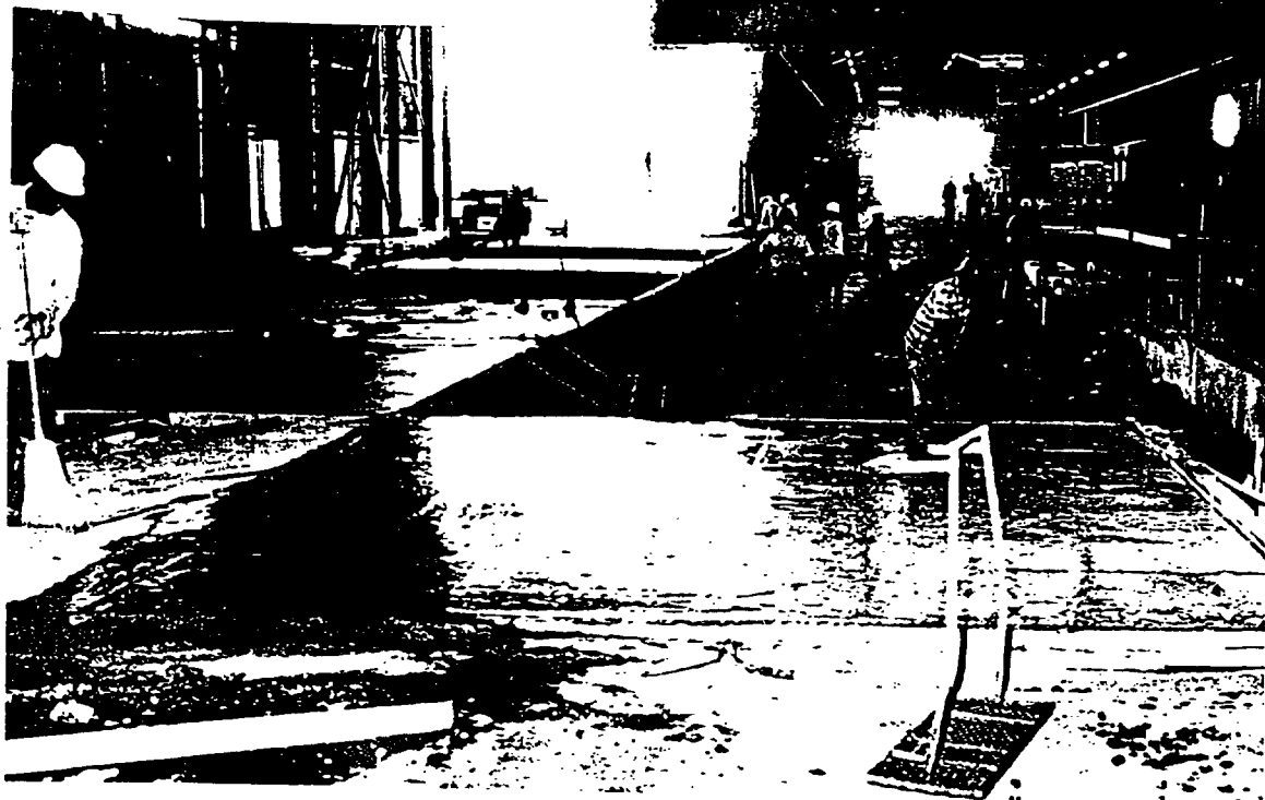
Floor Slab, Building 034 Looking South, 8-16-73
