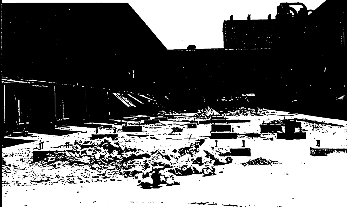
A-446 System Control, Building 60-D Looking South, Auth #731241 5-2-74
