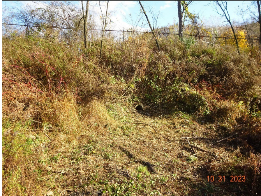
Photograph 33. DSC04864.JPG Description: Stormwater Outfall 017.
