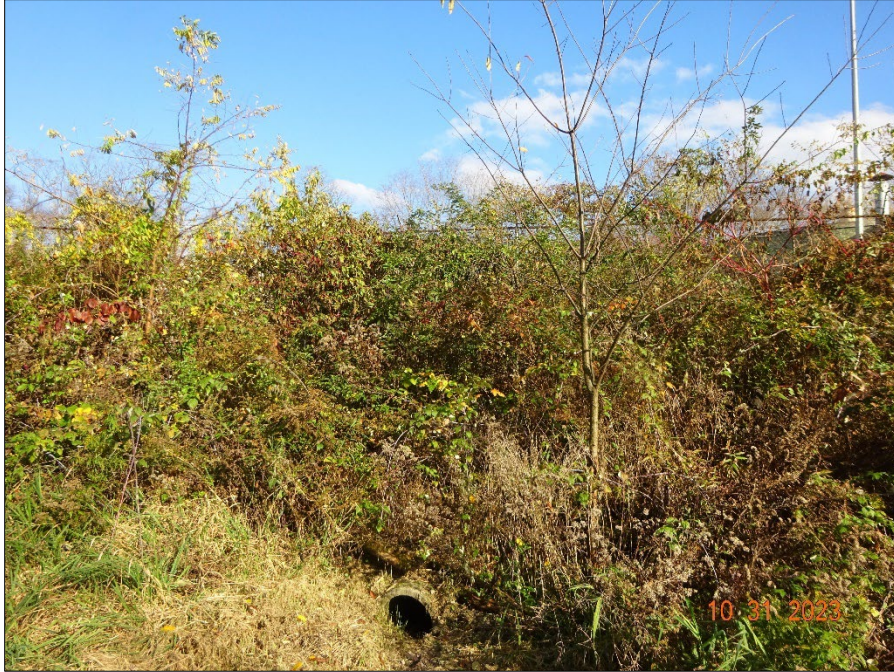
Photograph 31. DSC04862.JPG Description: Stormwater Outfall 015.
