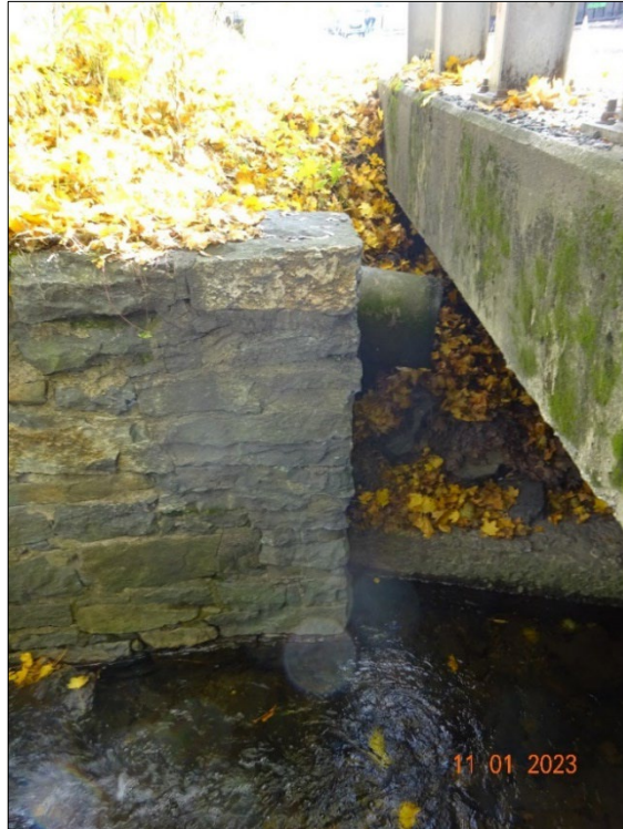
Photograph 42. DSC04917.JPG Description: CSO 009 anticipated location, the outlet was not able to be located.
