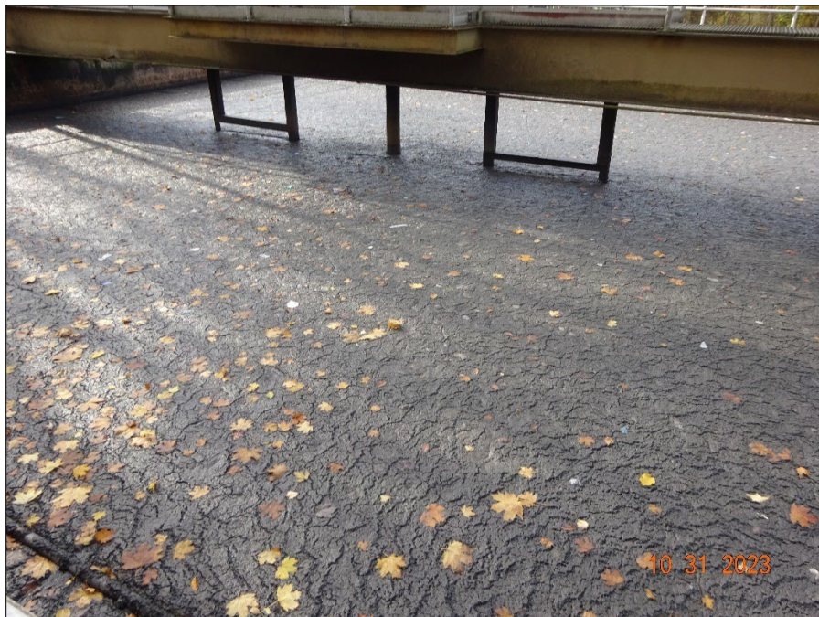
Photograph 14. DSC04784.JPG Description: Aeration Basin 2, currently being used for sludge storage and liquid decanting.
