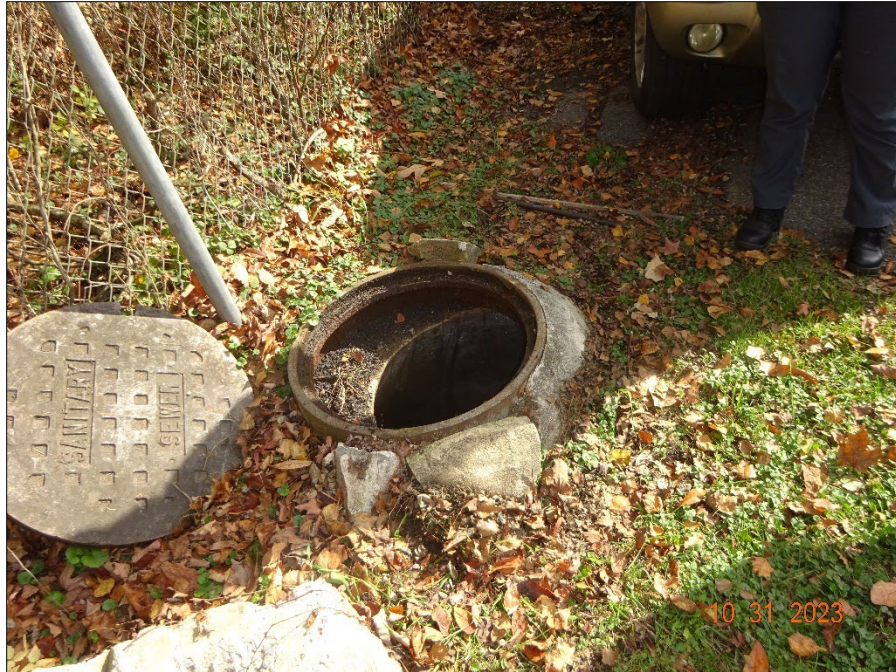
Photograph 1. DSC04746.JPG Description: Influent access manhole.
