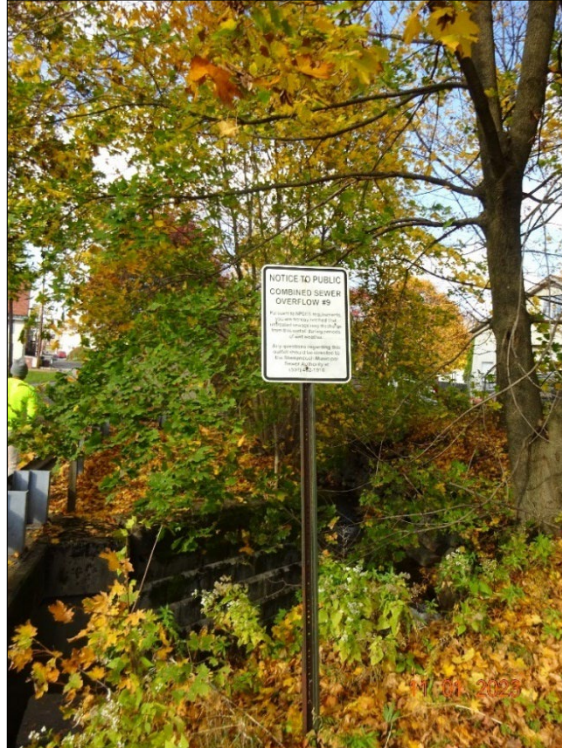
Photograph 41. DSC04916.JPG Description: CSO Outfall 009 signage.
