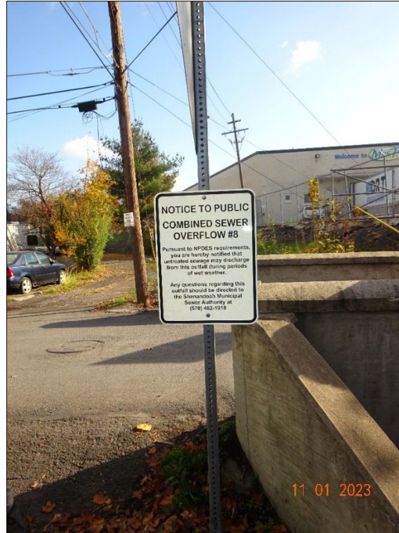
Photograph 39. DSC04902.JPG Description: CSO Outfall 008 Signage.
