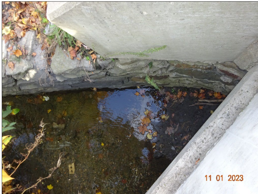
Photograph 40. DSC04904.JPG Description: CSO Outfall 008 anticipated location, the outlet was not able to be located.
