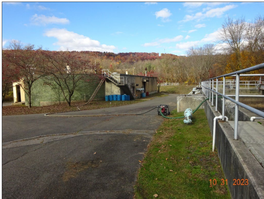
Photograph 16. DSC04785.JPG Description: Temporary transfer line to move contents of Aeration Basin 2 to the anaerobic digesters.
