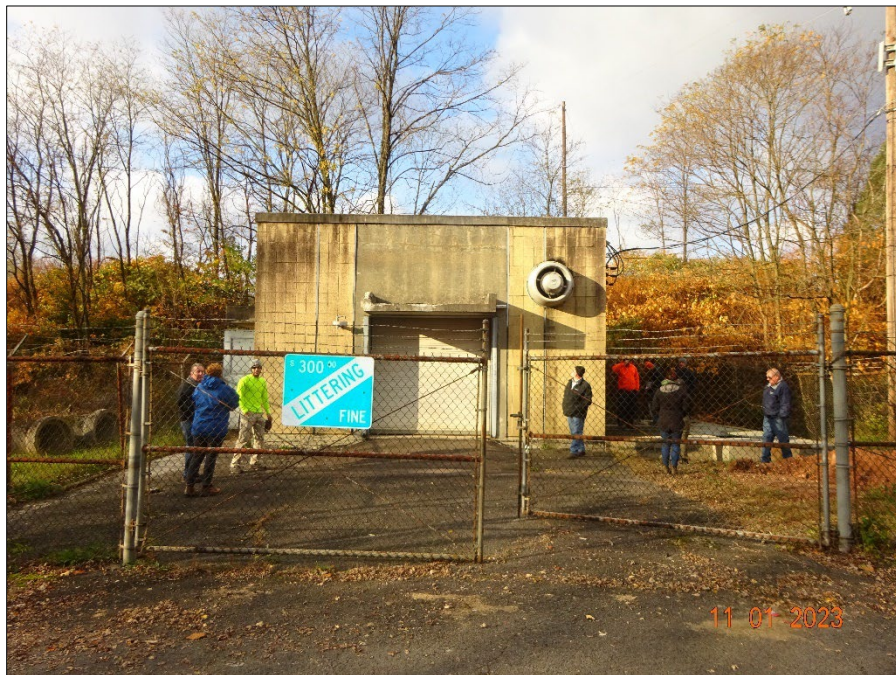
Photograph 34. DSC04873.JPG Description: Pump Station 1.
