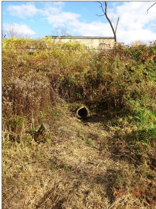
Photograph 32. DSC04863.JPG Description: Stormwater Outfall 016.
