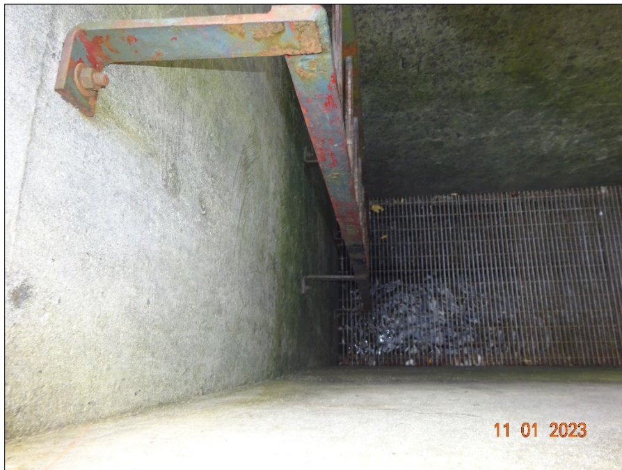
Photograph 36. DSC04875.JPG Description: Ladder to Pump Station 1 influent channel.
