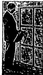
Cleaning Filter Elements with Portable Vacuum Cleaner
