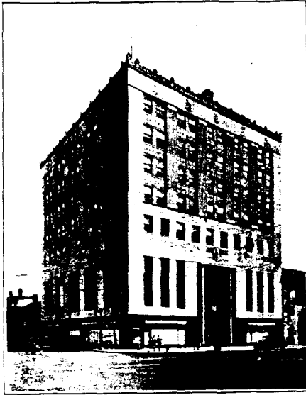
First National Bank & Trust Co. building in Hamilton, Ohio
