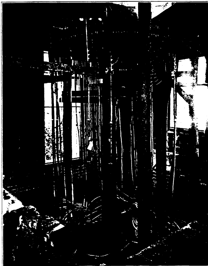
THIS WATER DIVIDER AT BRATTLEBORO, VERMONT, IS A MAZE OF LEAD PIPE
