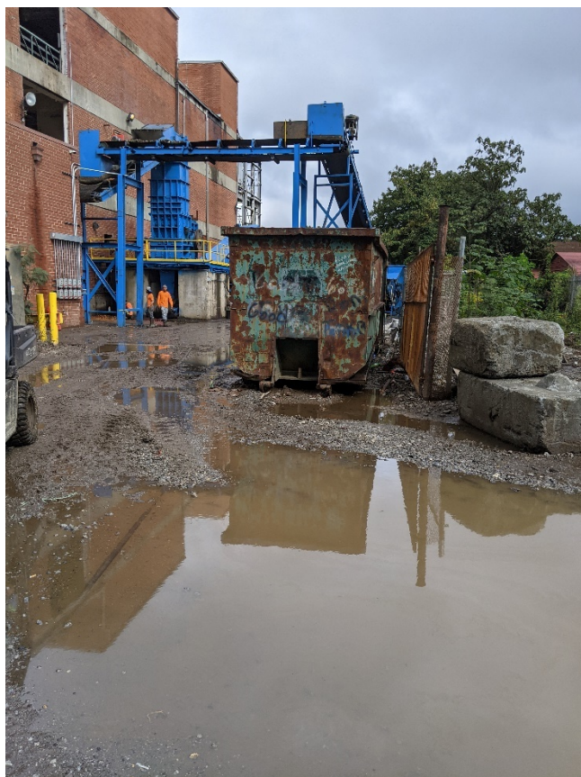
Figure 85: PXL_20211006_152327728.jpg – Plugged up Stormwater drain
