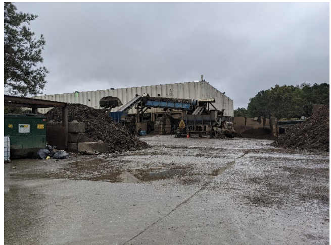
Figure 48: PXL_20211006_140722625.jpg – Receiving Area
