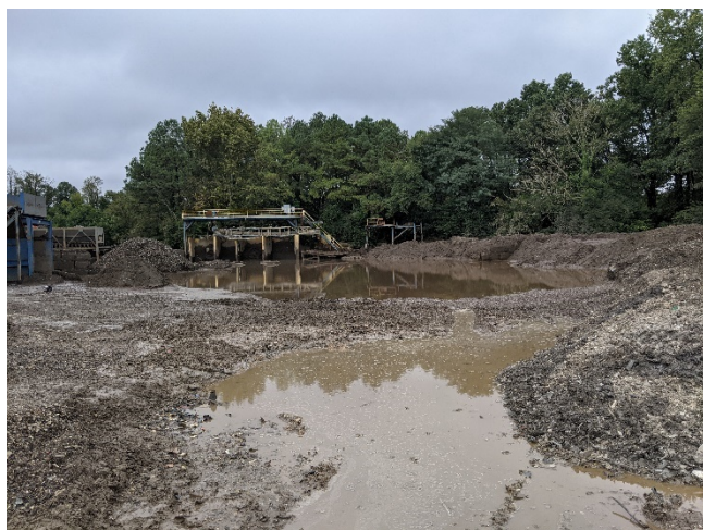
Figure 87: PXL_20211006_153116223.jpg – Receiving Area
