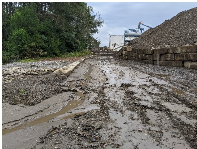
Figure 101: PXL_20211006_181402496.jpg – Wastewater flow approaching Outfall 3
