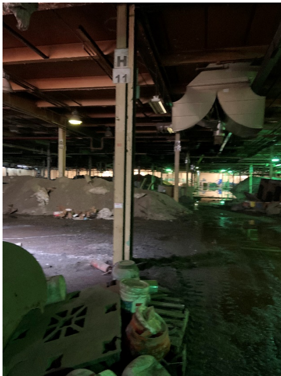
Figure 35: IMG_3104.jpg – Piles of solid waste stored in the Keebler Building
