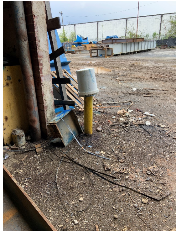
Figure 12: IMG_3081.jpg – View from rear of Fabrication Building
