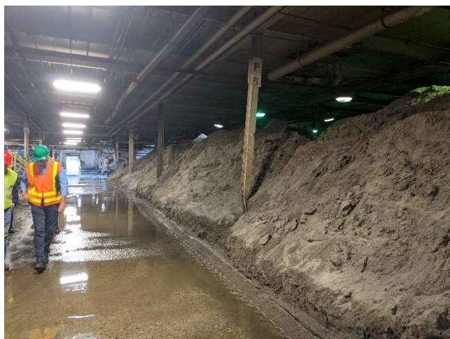
Figure 61: PXL_20211006_145612675.MP.jpg – Solid Waste stored near the Waste Water Treatment area
