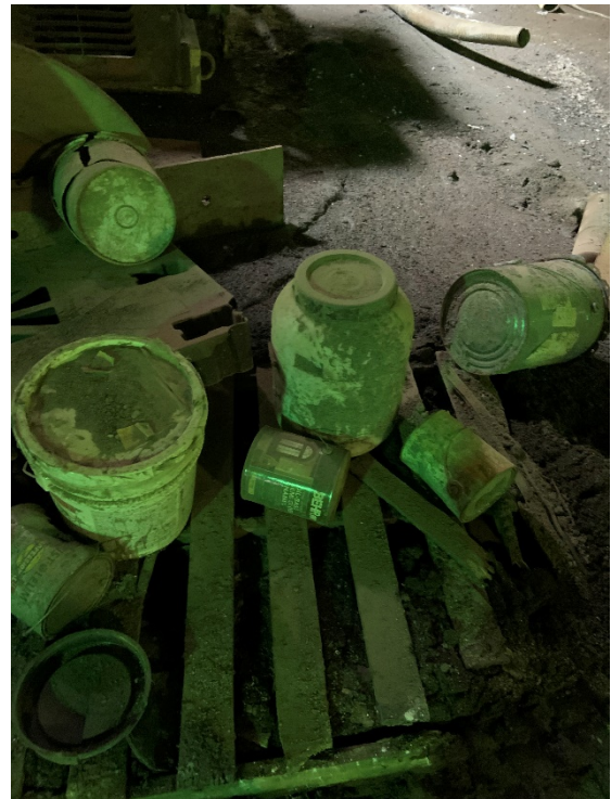
Figure 40: IMG_3109.jpg - Containers of unknown waste in the Keebler Building
