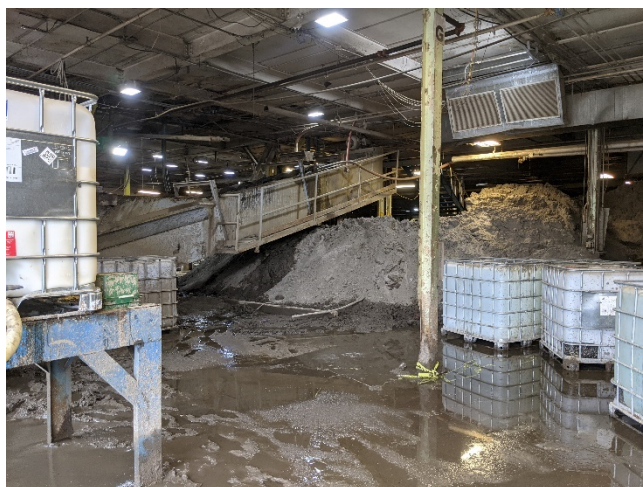
Figure 70: PXL_20211006_150131436.jpg - Wastewater Treatment Area
