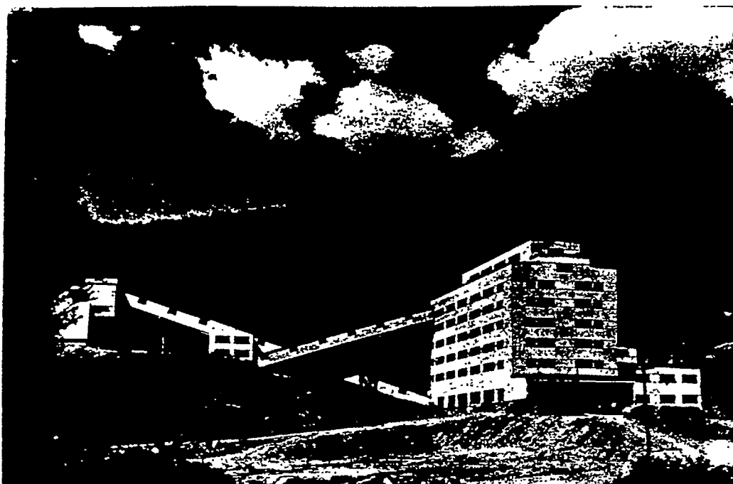
FIGURE 13.--Mill of Vermont Asbestos Mines Near Eden, Vt.
