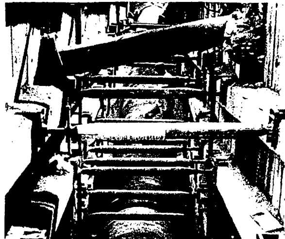
Deep trenches in some soils require shoring and sheeting.
