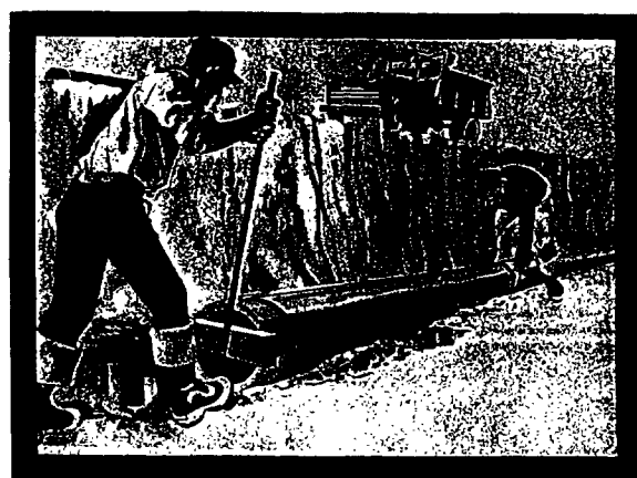
Fig. 18. Method of pushing pipe lengths together.
