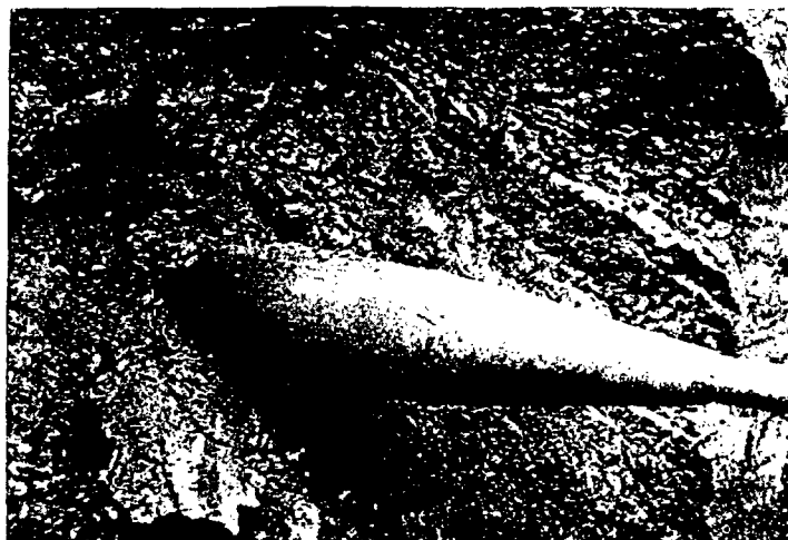
Tunneling mole for service line installation.
