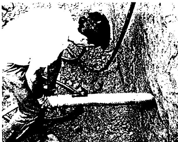
Tunneling mole for service line installation.
