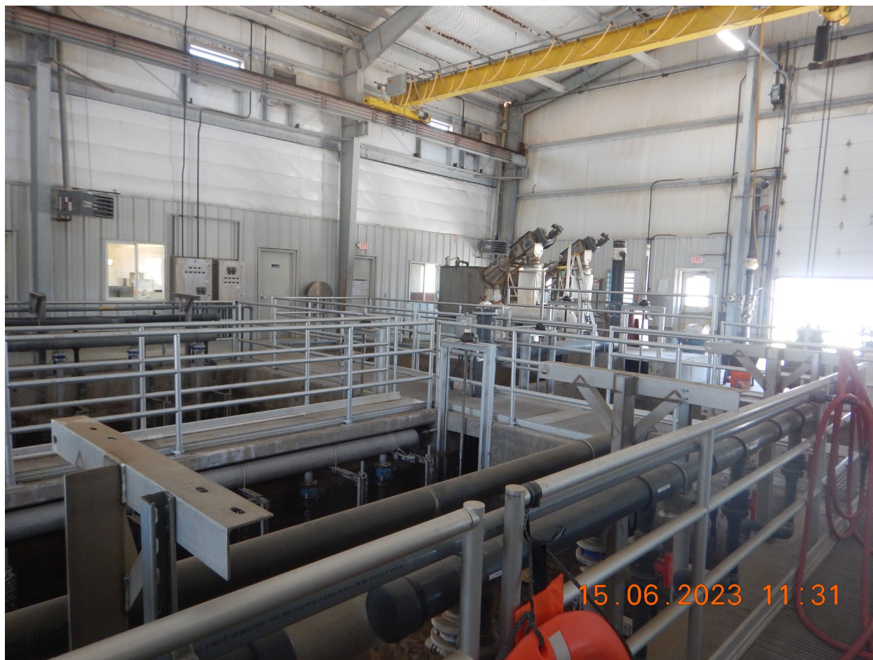
View of the MBR basins and headwork structure looking approximately Northwest. (DSCN 2590). Photographed by D. Esparza.
