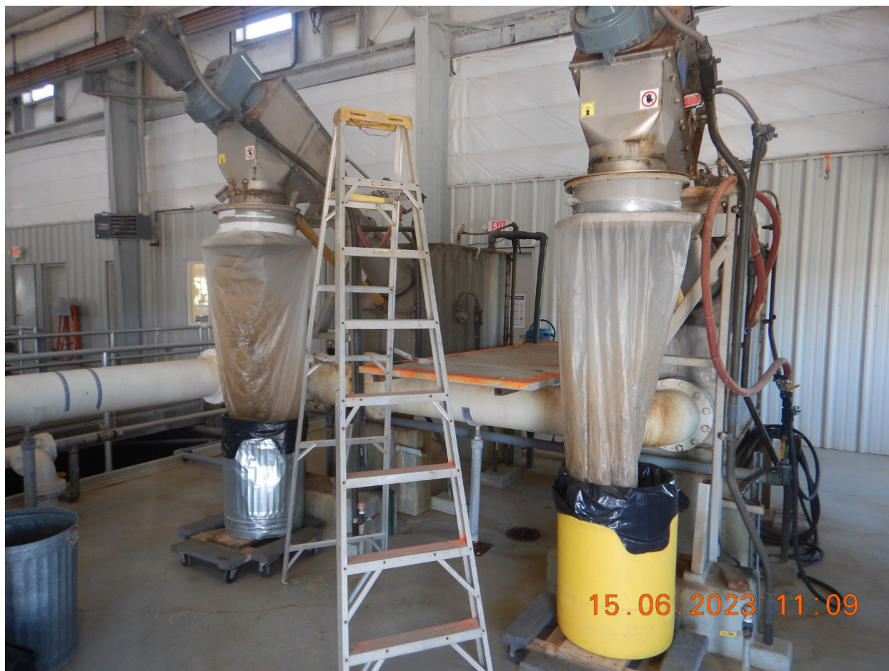
Picture of San Felipe WWTP Headworks structures. (DSCN 2587). Photographed by D. Esparza.
