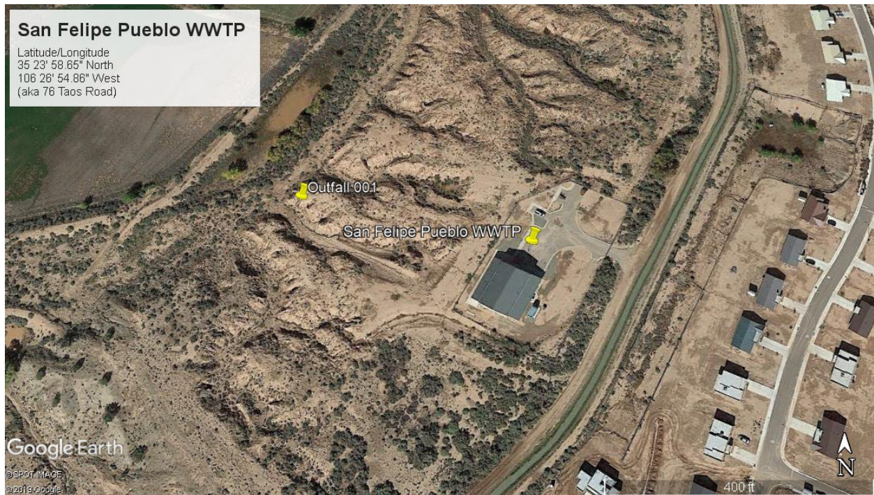
Aerial Image #1: Overall view of the San Felipe Pueblo Wastewater Treatment Plant location and the approximate location of Outfall 001. Aerial from Google Earth Maps.
