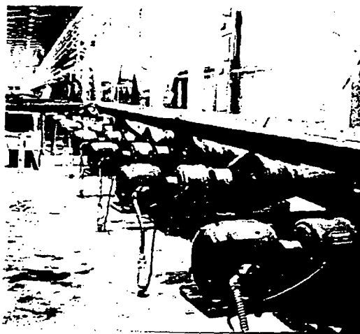
This pipe conveyor is driven by a line of Elliott C-W 1-hp, 1800-rpm enclosed induction motors.
