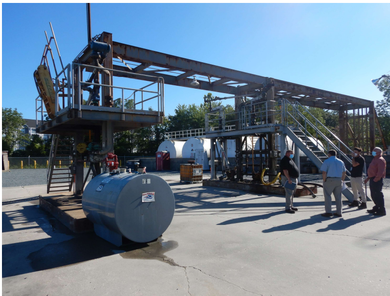
DSCN2463 View of Facility Filling Station
