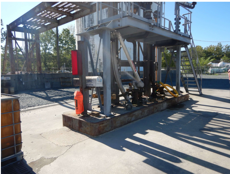
DSCN2466 View of Filling Station
