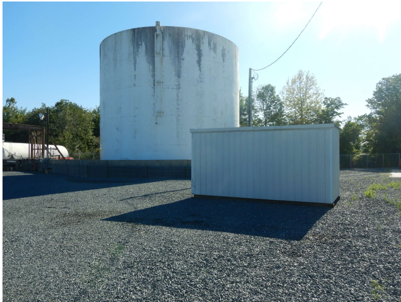
DSCN2462 View of decommissioned 500,000-gallon storage tank
