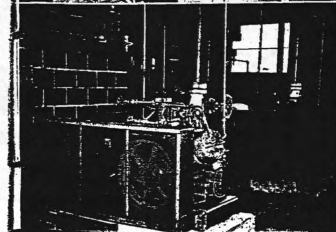
Above left—The Worthington compressors at the Amherst rink are driven by two 75-hp Elliott C-W motors. In the foreground of the picture can be seen two Elliott Crocker-Wheeler 20-hp motors being used as pump drives.
