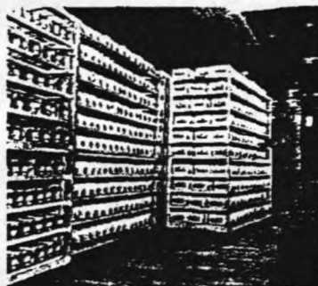
These racks of bread are being quick-frozen at 20 degrees below zero in the quick-freezing room of the new refrigeration and storage plant of Arnold Bakers, Inc., Port Chester, N.Y.
