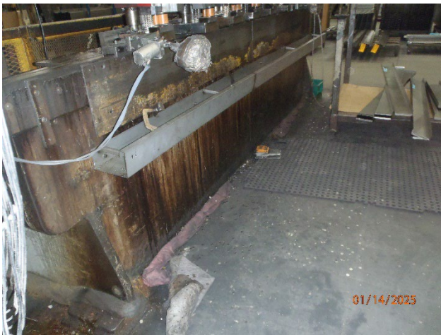
Picture 2 – Press brake machine oil release
