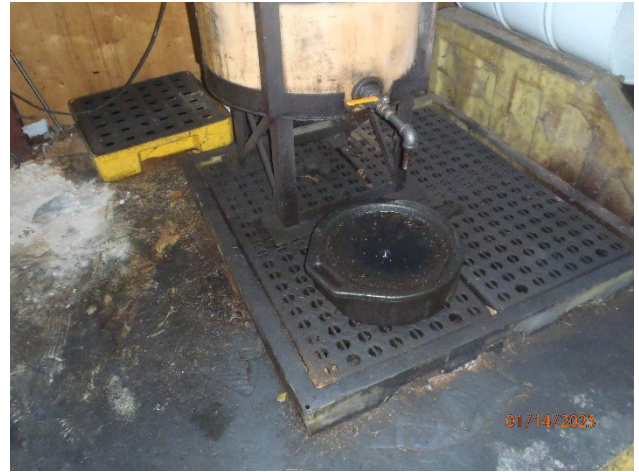
Picture 4 – Used Oil Drum Storage unmarked secondary containment
