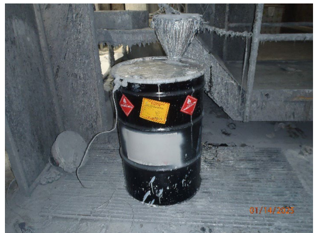
Picture 29 – Paint Area Filter Wall SAA
