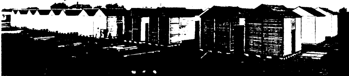
Typical group of Nebraska's white lead painted AAA grain storage bins.
