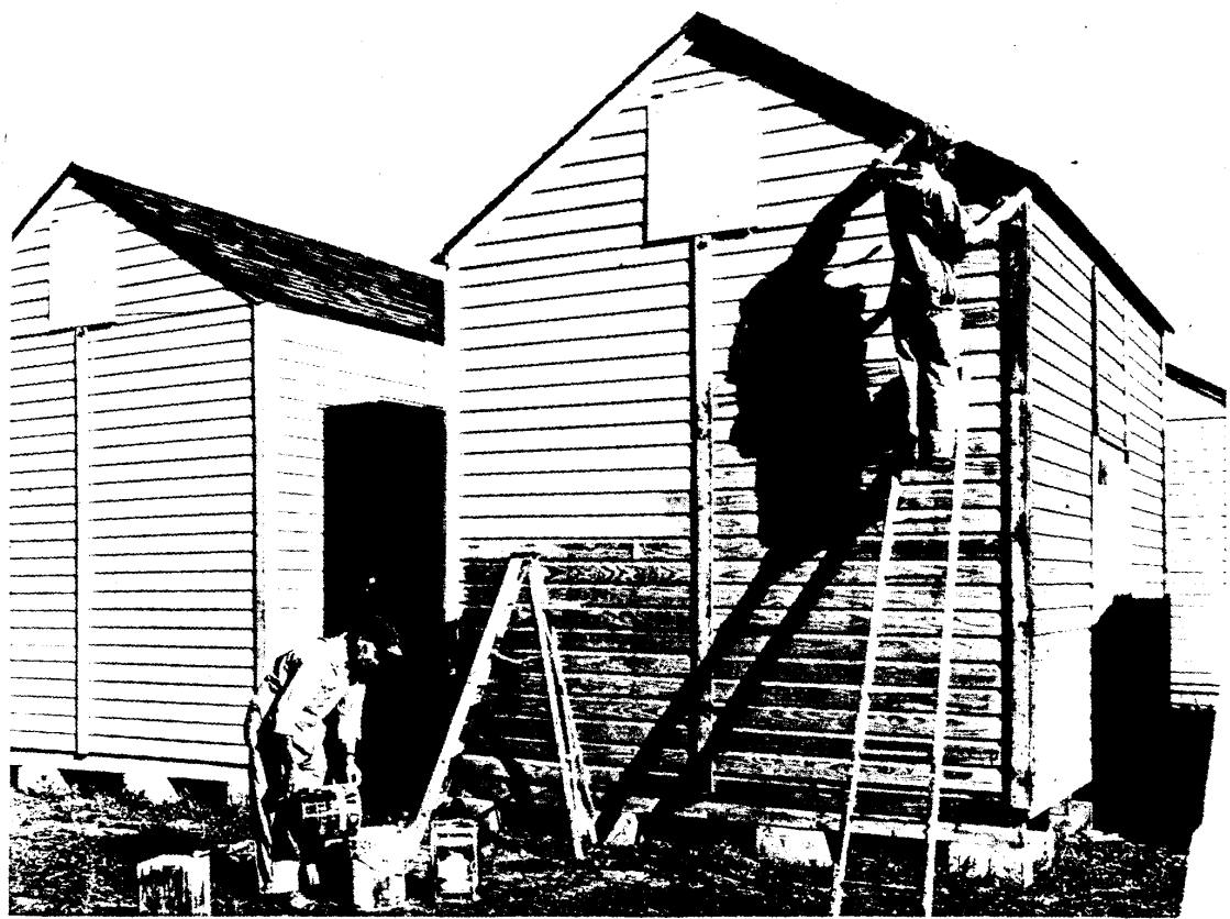
Applying priming coat of pure white lead paint to grain storage bins at York, Nebraska. 4,000 of these bins erected by the Nebraska Agricultural Conservation Committee will be painted with pure white lead paint.
