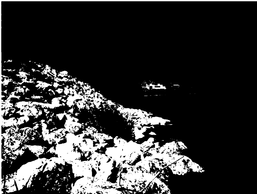
Photo 2. Overview of northwest end of rip-rap, taken from bottom of rip-rap (facing northwest)
