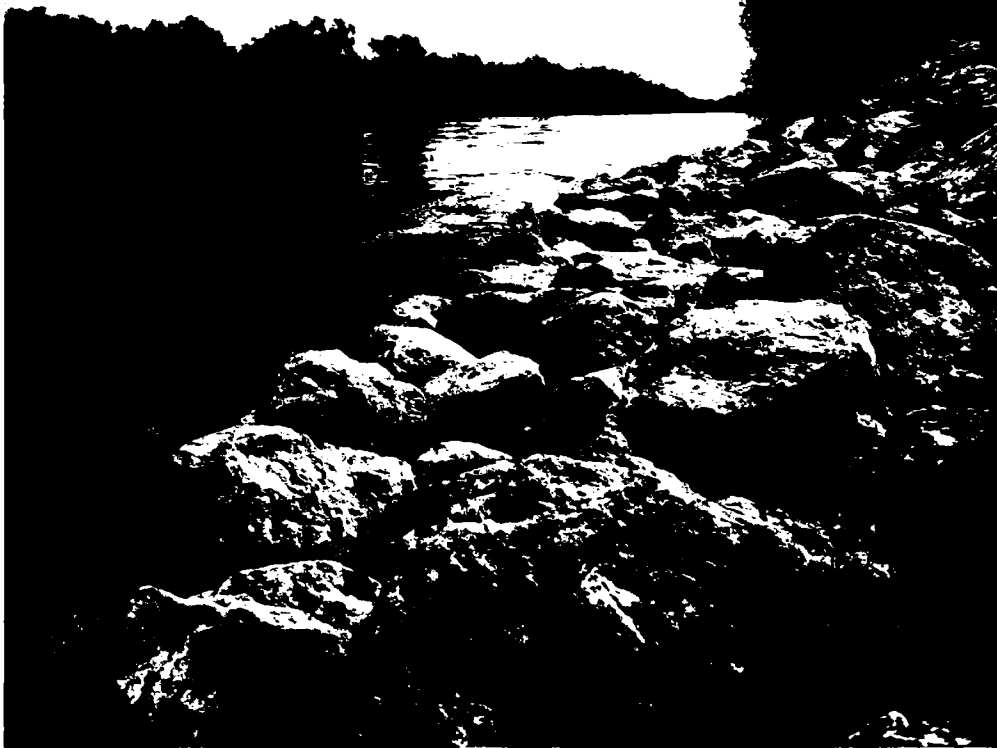
Photo 3. Overview of southeast end of rip-rap, taken from bottom of rip-rap (facing southeast)
