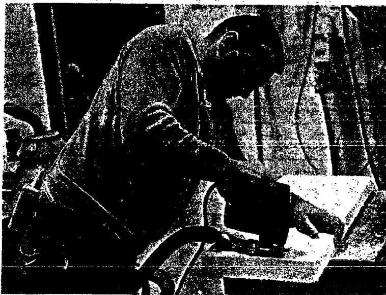
Charles Collins, President of Local 30 of the Asbestos Workers Union, cutting calcium silicate block during the powered hand-saw trials at the Hoffman Air Systems plant in Syracuse, New York.
