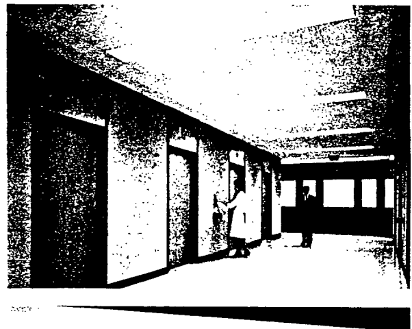
CENTRAL CORE , housing high-speed elevators and building services, was fireproofed with PYROBAR gypsum tile (above), plastered and covered with different colors of vinyl fabric on alternate floors (at right). Floors and beams were fireproofed with FIRECODE "V".
