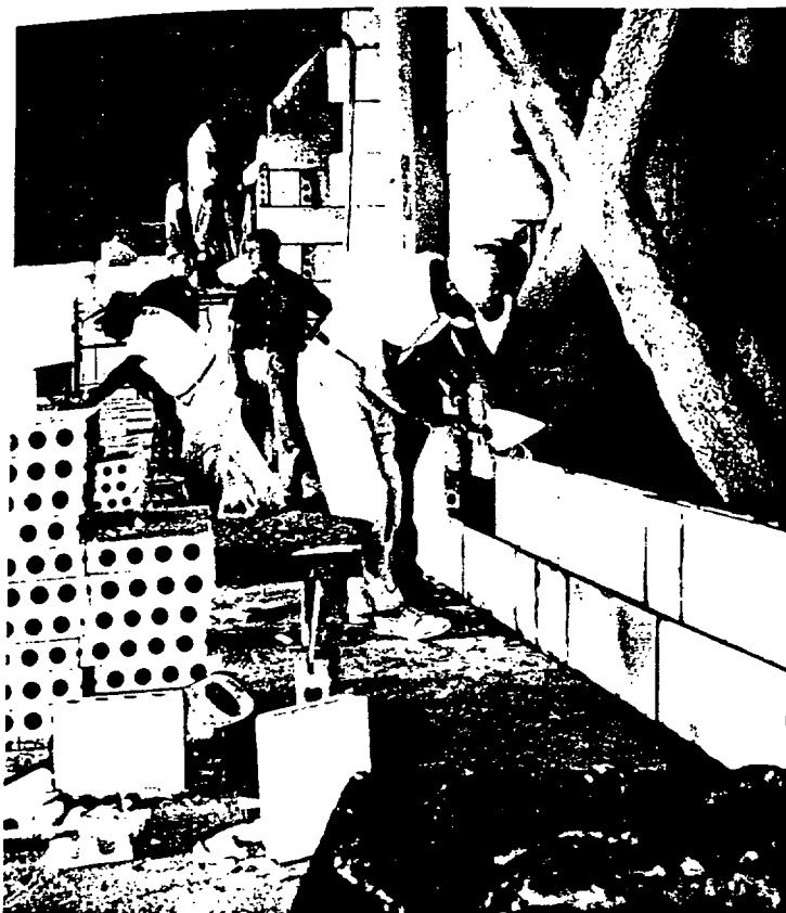
CENTRAL CORE , housing high-speed elevators and building services, was fireproofed with PYROBAR gypsum tile (above), plastered and covered with different colors of vinyl fabric on alternate floors (at right). Floors and beams were fireproofed with FIRECODE "V".
