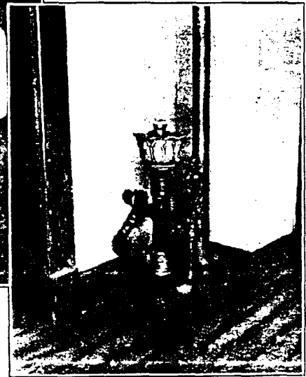
Lavatory with untrapped waste direct to sewer. The fountain bowls at left and right are old light globes.
