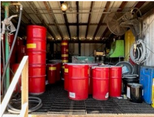
Photo #9 – Containers in the Drum washer/storage tanker dumpster unit.
