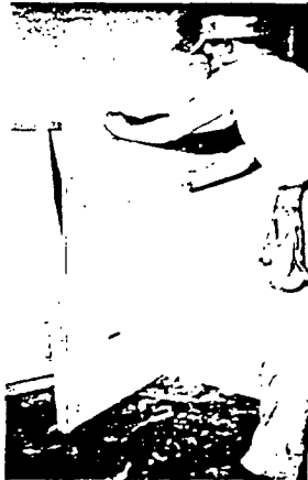
Break the gypsum core of SHEETROCK by snapping and bending away from the scored paper side. Complete cutting by running knife through back paper from above or below.
