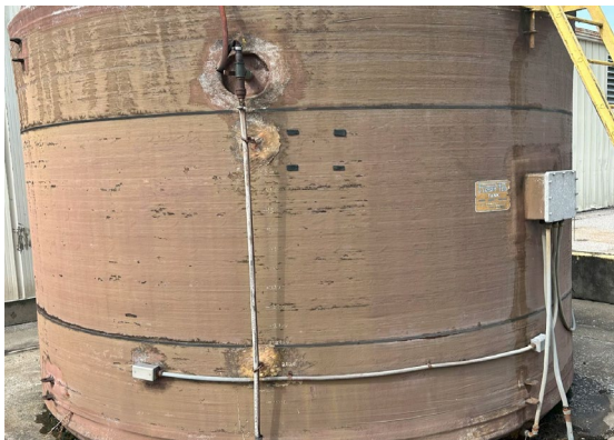
Photo-5 7,500-gallon Unlabeled Used Oil Tank
