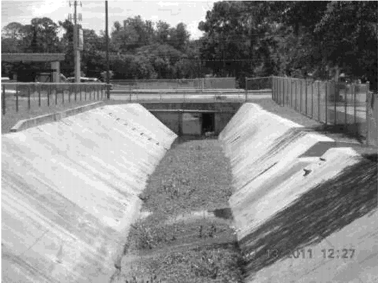
Figure 16: Pinellas Park Ditch #5 discharges directly into a wetland that discharges into “Joe’s Creek.” Joe’s Creek is currently a water of the United States. The park ditch is a conveyance managed as part of the Pinellas Park Water Management District, which was created in 1976 by the Florida State Legislature to manage the primary stormwater drainage/flood control system for a portion of central Pinellas County. The ditch provides no environmental or human benefits, other than flood control. It is not now considered to be a water of the United States, but would be considered to be such under the proposed rule. 463
